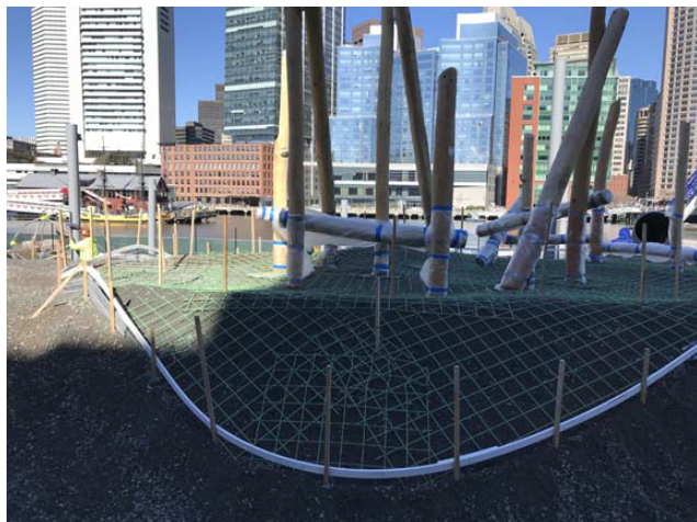
Form work for slab under log climber
