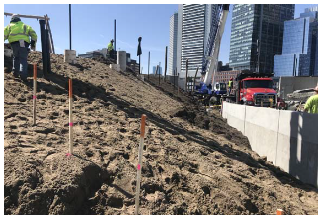
Planting soil installation
