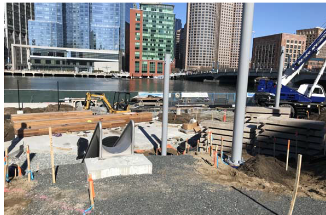
Shade structure post install
