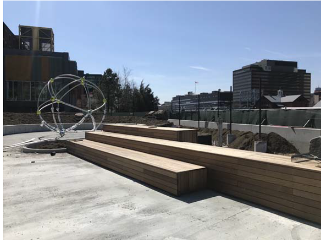
Mud slab at amphitheater
