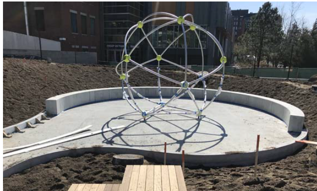
Mud slab at Cosmo climber
