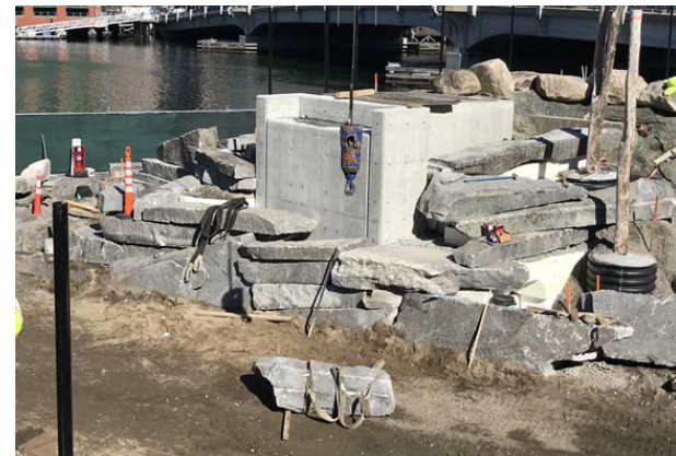
Stone tailing wall progress
