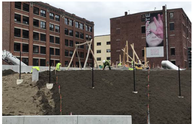
Planting soil and fence post installation
