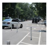
**Added daylighting at intersections** to open up sight lines at corners.
