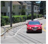
Used pavement markings and flex posts to better guide vehicles through a curve approaching the intersection on Wood Avenue near Mariposa Street in Mattapan.
