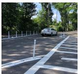
Installed temporary curb extensions using pavement markings and flex posts at New England Avenue and Southern Avenue in the Talbot Norfolk Triangle.
