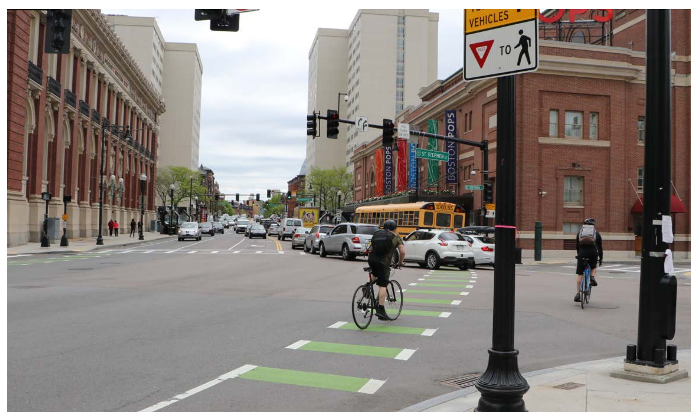
Marked bike crossing (Massachusetts Ave.)
