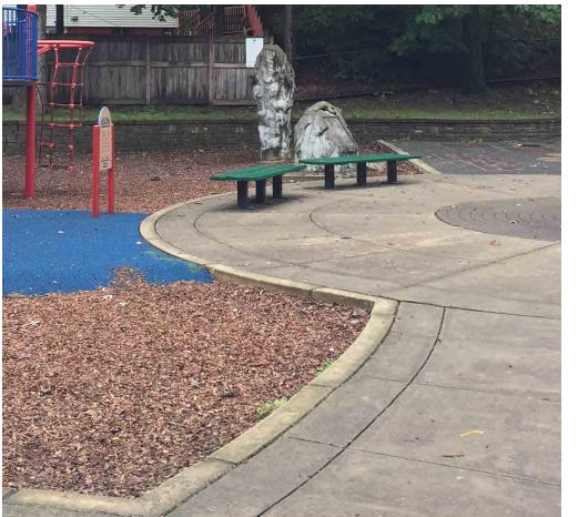
Concrete curbs are located between paths and existing play areas with +/- 6 inch difference in elevation. All walkways are concrete except for the painted asphalt play areas and brick accents in the center of the circle.
