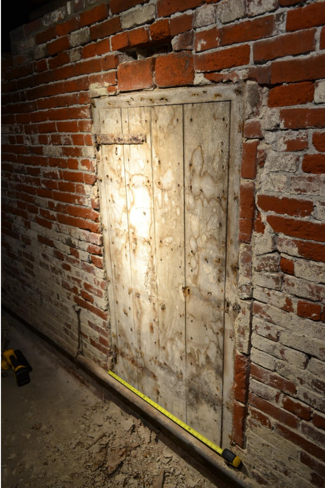
Figure 23- Tomb 12 door after removal of mortar, metal mesh, and lathe. Exposed yellow portion of Measuring tape is 75 cm in length.
