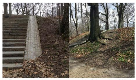
Stairs near pond with erosion alongside sluice and social trail stripped of vegetation
