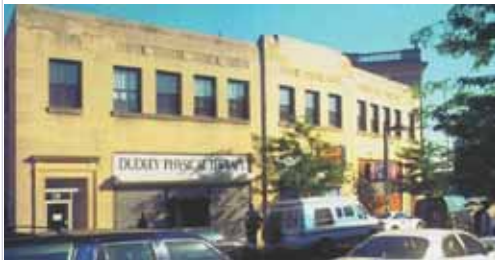
Before view of Roxbury storefront
