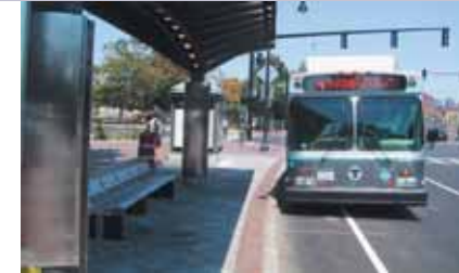
Washington Street bus shelters & street furniture
