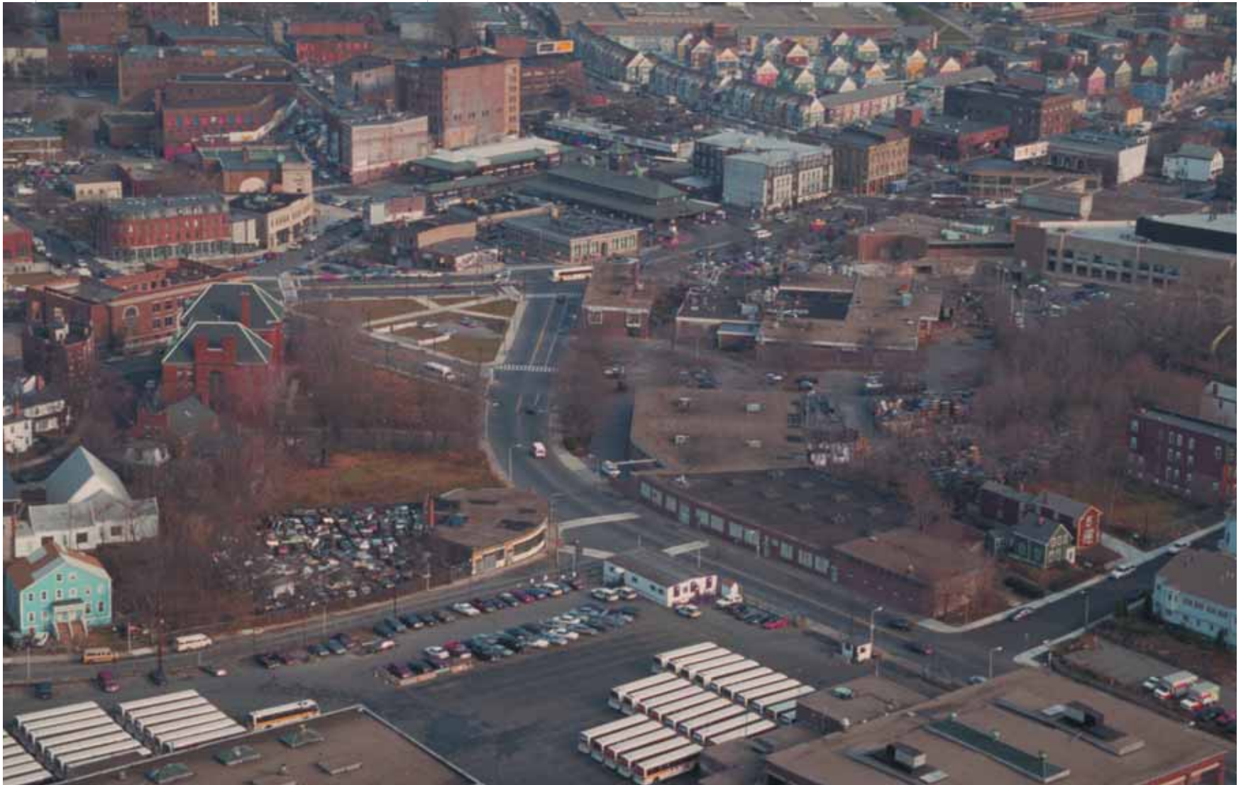
Aerial view of Dudley Square
