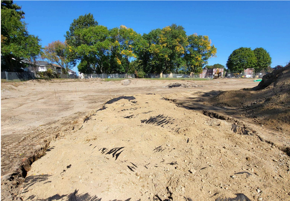
Underground stone pocket drainage system being installed in the field area.
