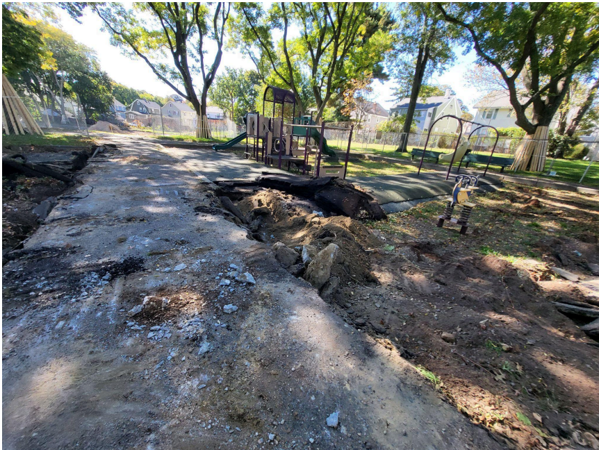
Playground demolition in process.
