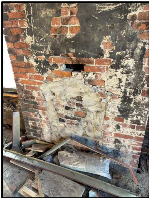
Figure 2c (left) Sixth floor chimney with missing and damaged brick construction Figure 2d (right) Sixth floor brick wythes delaminating from each other at interior
