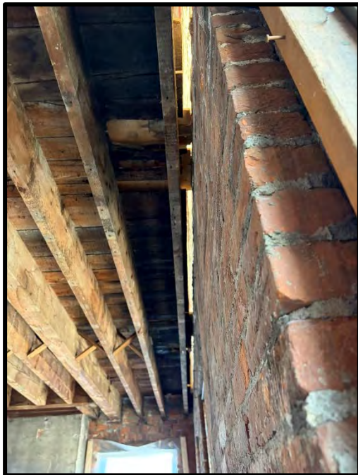
Figure 3a (left) Existing joists with gap visible at west façade
