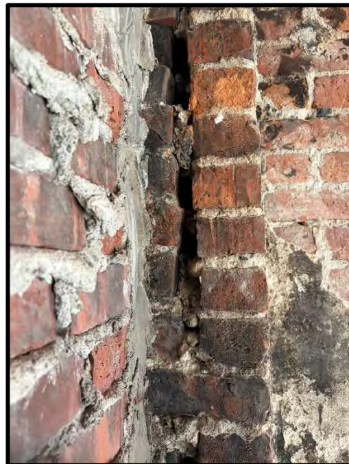
Figure 2c (left) Sixth floor chimney with missing and damaged brick construction Figure 2d (right) Sixth floor brick wythes delaminating from each other at interior
