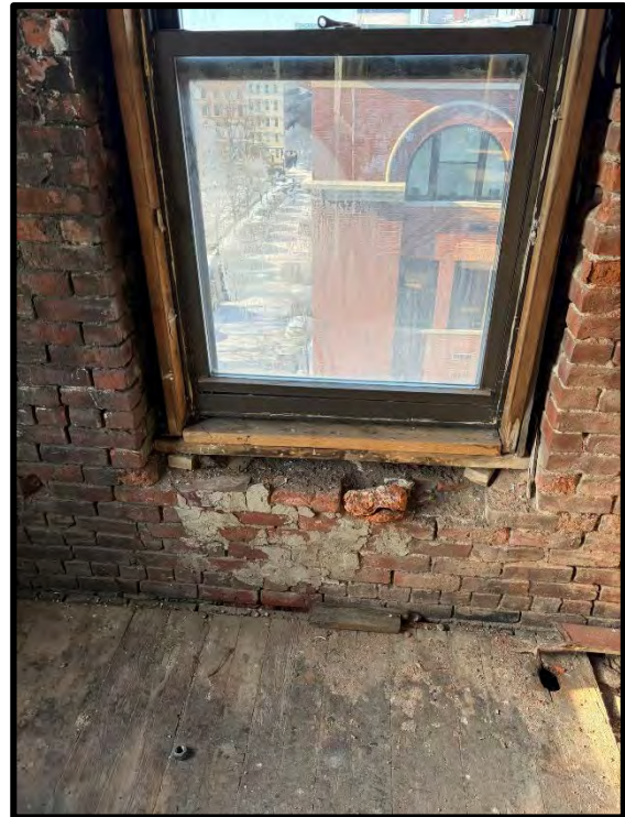
Figure 2a (left) Sixth floor interior façade and window header. Open mortar joints and loose brick visible Figure 2b (right) Sixth floor window sill with missing brick, loose and displaced brick and missing mortar
