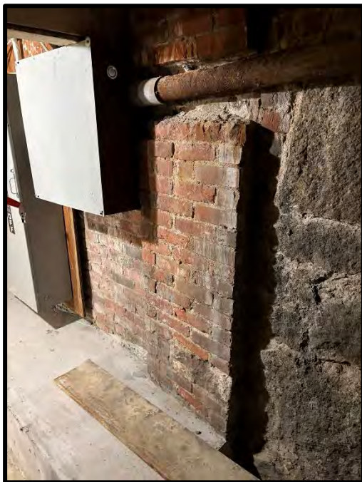
Figure 4b (left) Brick masonry foundation wall Figure 4c (right) Brick pier in basement
