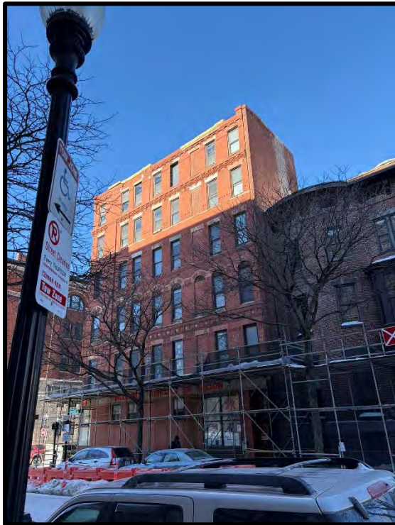
Figure 1c (left) South façade parallel to Shawmut Avenue
