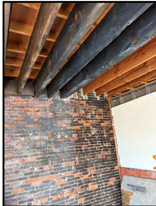
Figure 2f (right) Interior west façade at third floor showing gap between façade and third floor framing
