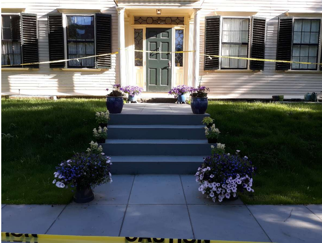
Ex. Bluestone terrace and stairs, in foreground.
