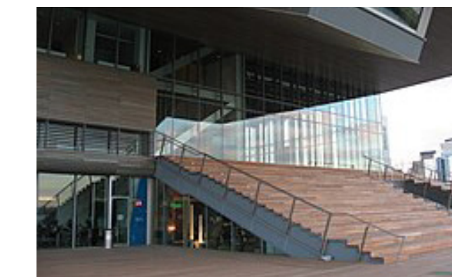
ICA STEPS/ ESCALERAS ~0.5 ACRES
