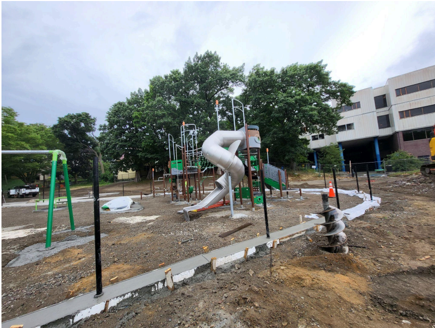
New 5-12 playground structure has been installed.
