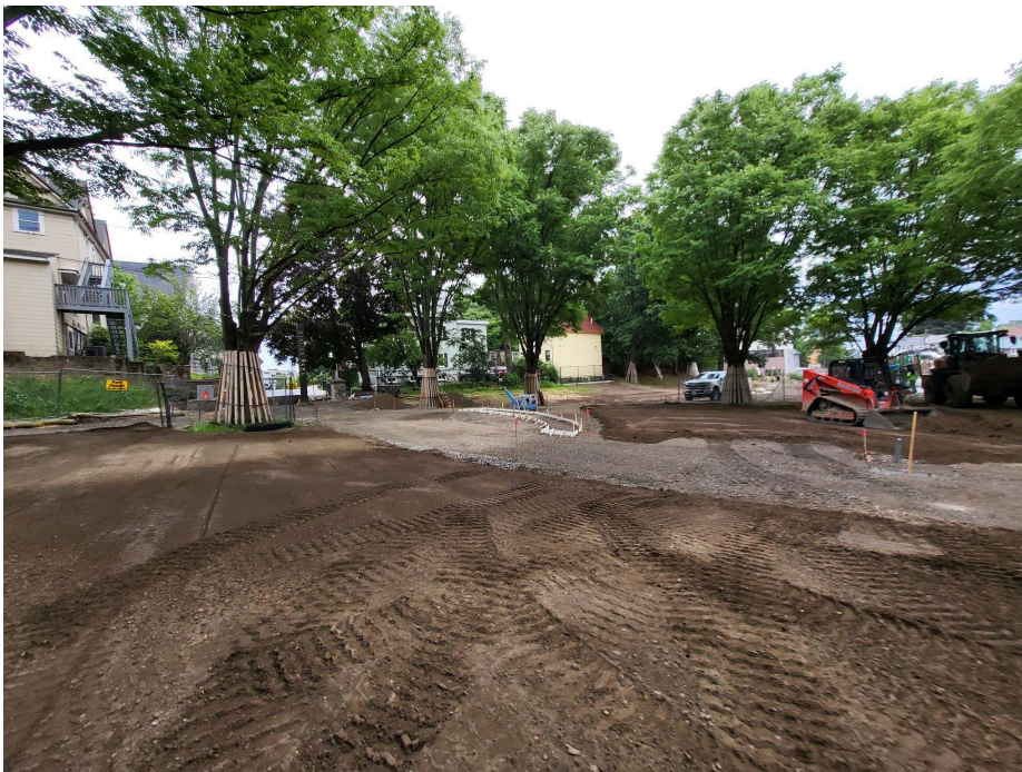
The gathering area is being graded and seeded.
