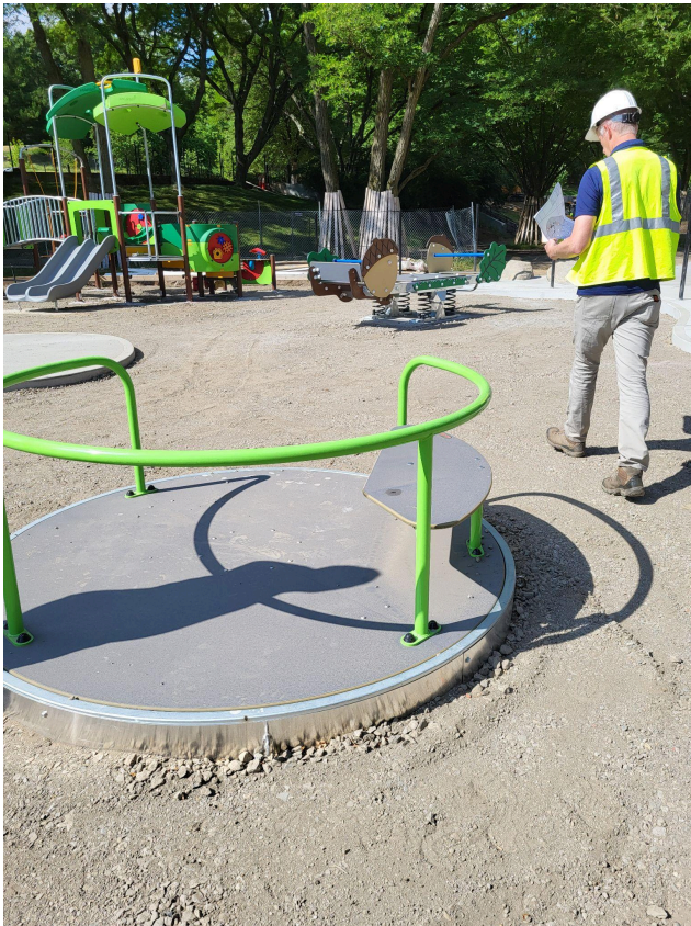
The new accessible spinner has been installed!
