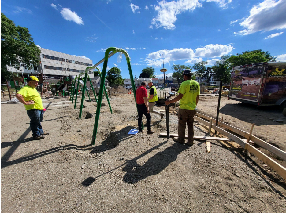
New swing bay is being installed.
