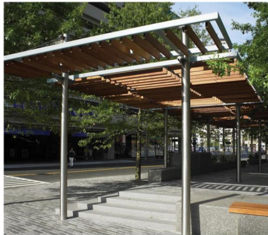
Open Shade Structure
