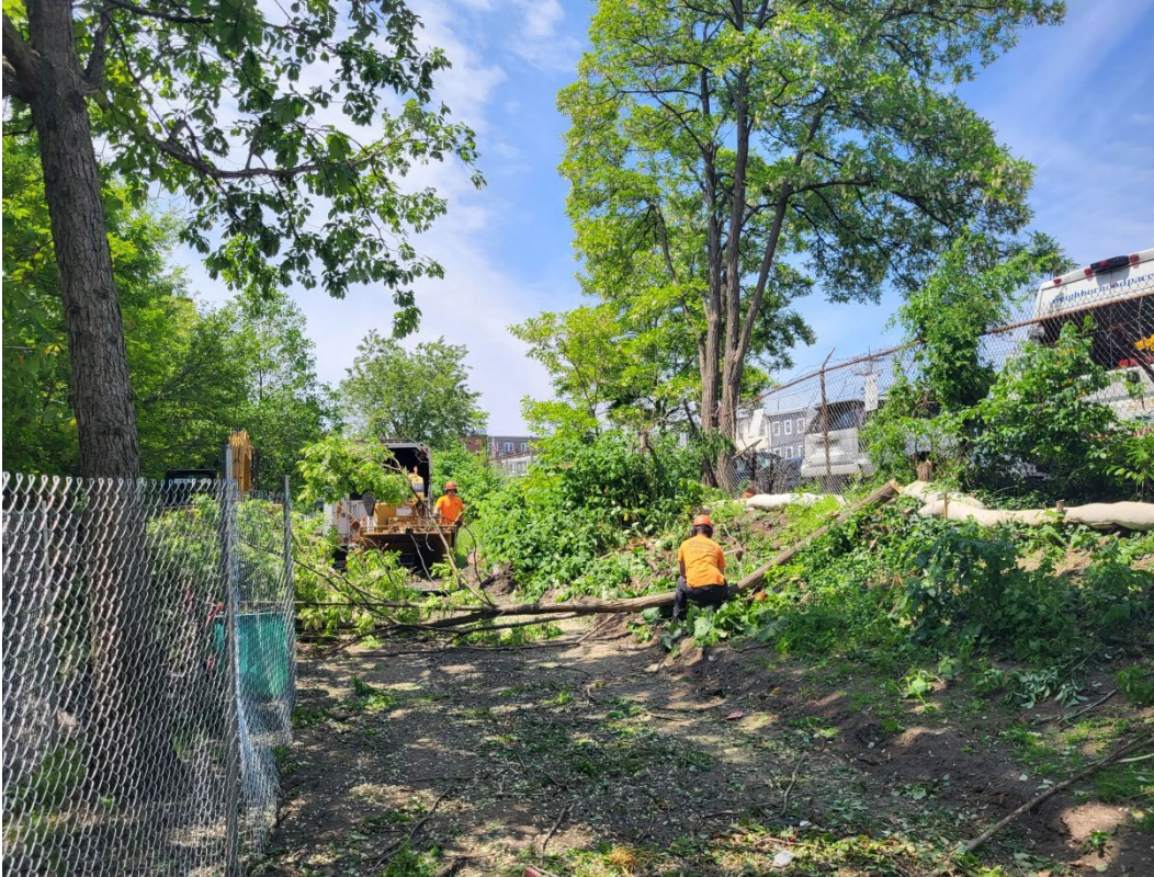
Ongoing removal of dead, dying and invasive trees
