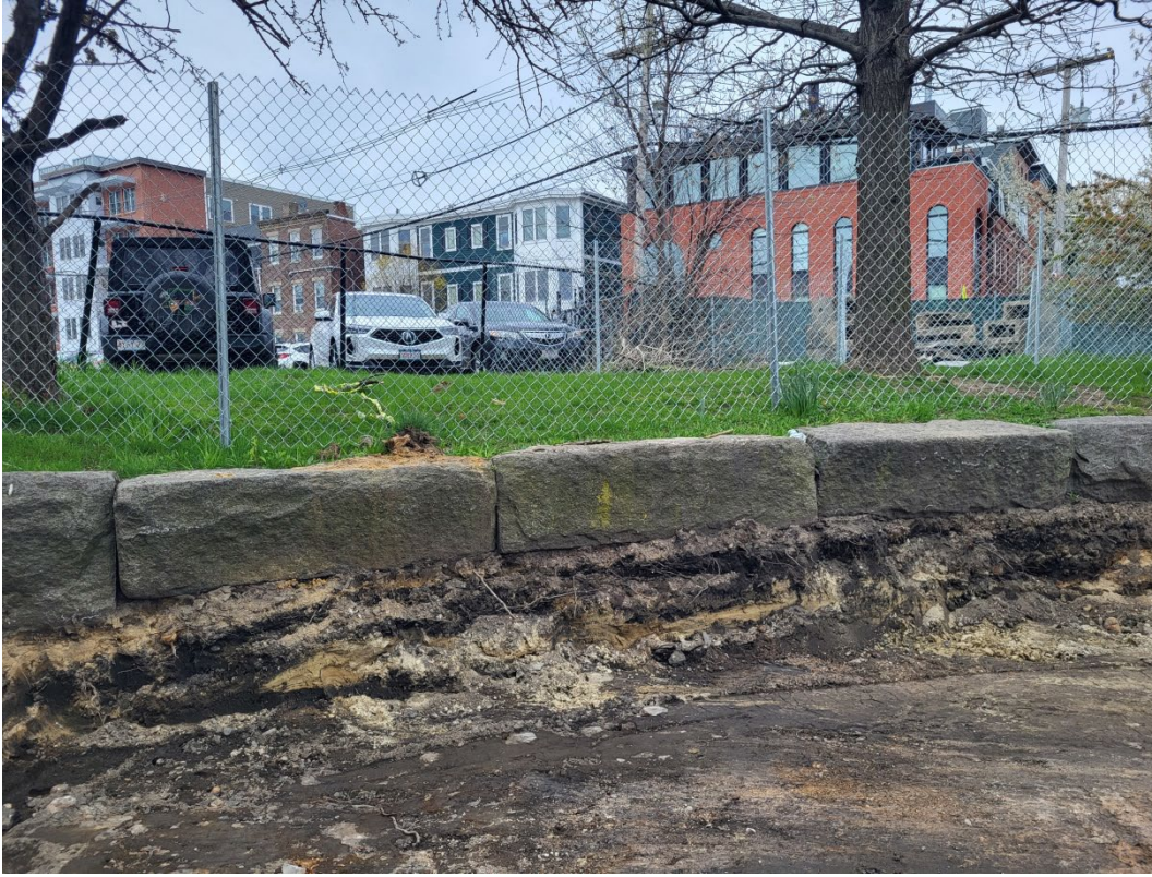
Block wall and plaza area at Gove Street (photo above and below) A row of granite blocks will be added to address the change in elevation
