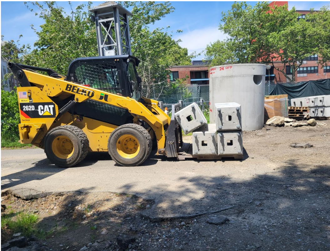
Additional light pole footings were delivered this week
