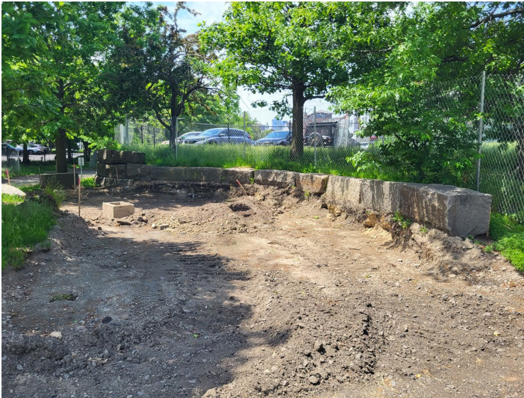
Block wall and plaza area at Gove Street (photo above and below) A row of granite blocks will be added to address the change in elevation
