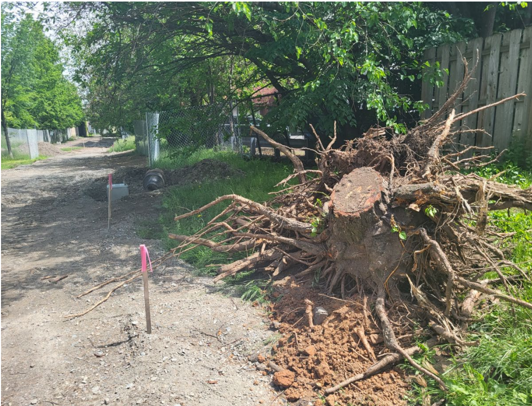
Tree roots from removed trees
