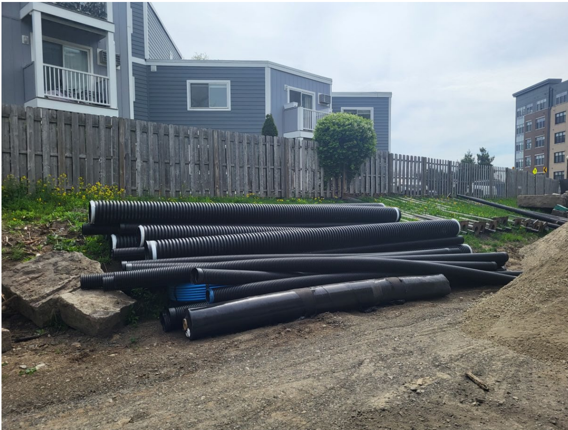
Drain pipes being store on site prior to installation
