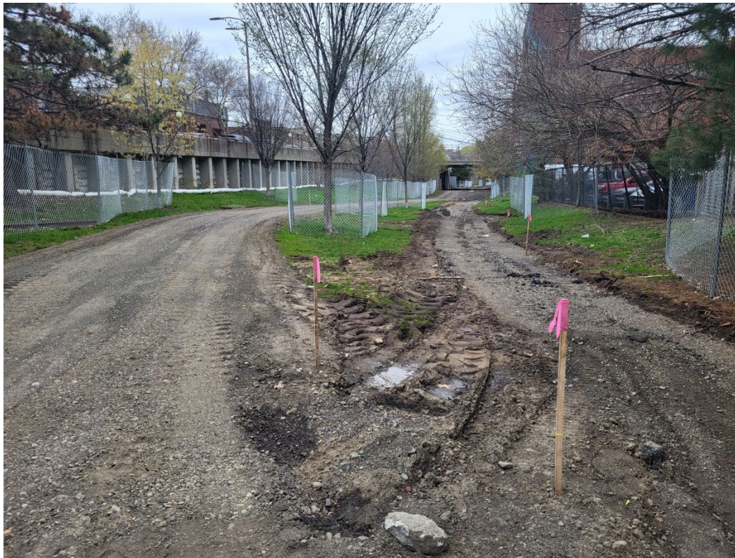
Completed demo of the asphalt path
