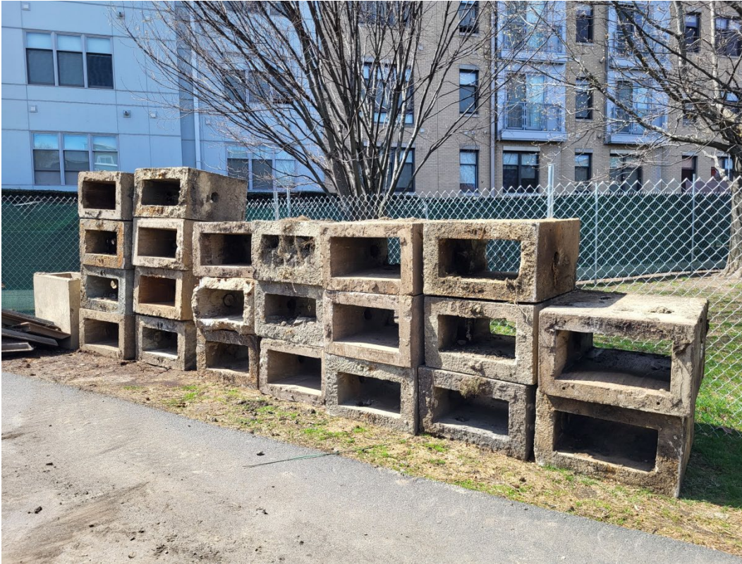
Stockpiled salvaged electrical handhole boxes
