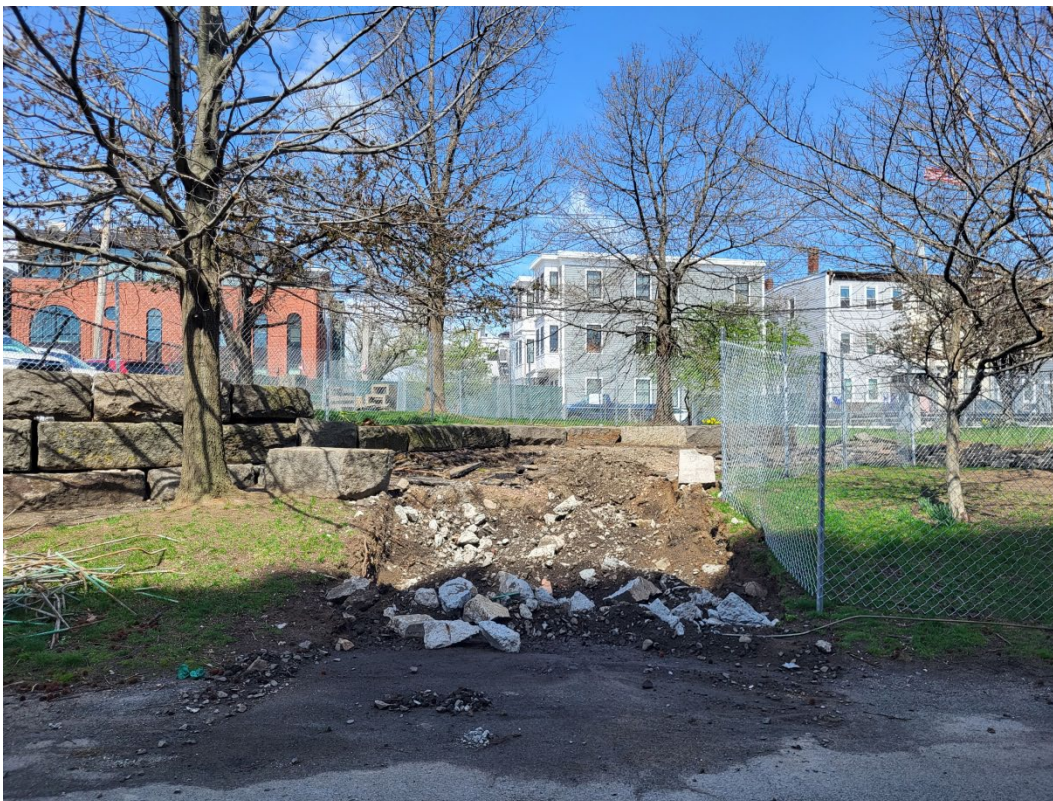
Demolition of the stairs at Gove Street
