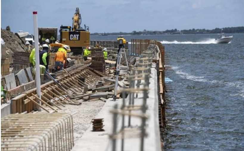
Outboard Floodwall Construction, Charleston, SC
