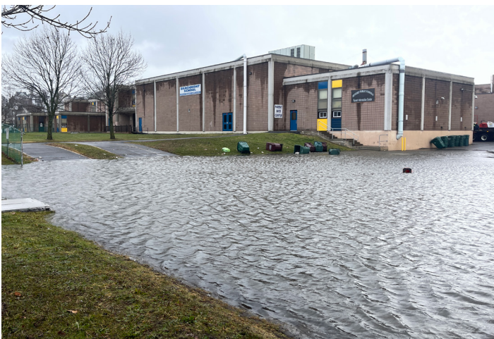
Flooding at the Beachmont Memorial School parking lot in Revere.
