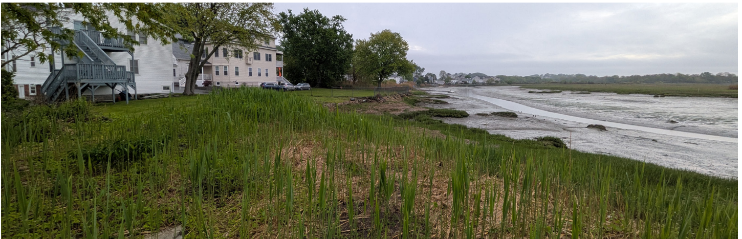
Residential Revere waterfront existing conditions, facing southeast.
