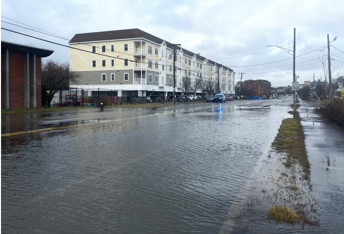
Flooding overtopping Bennington Street, looking northbound towards Revere.
