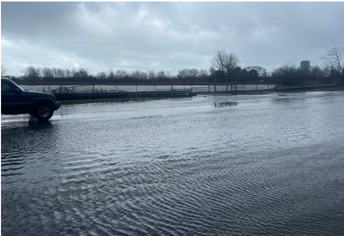
Flooding overtopping Bennington Street, looking at Belle Isle Marsh.
