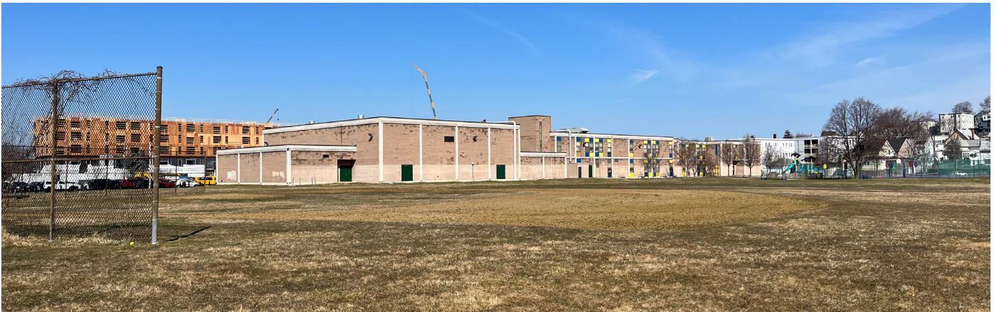
Fredericks Park existing conditions, facing the Beachmont Memorial School.
