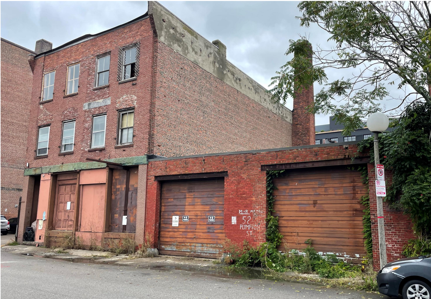
Figure X: Front facade of 52 & 56 Plympton Street. Note the following critical conditions that diminish the building's architectural and structural integrity: The removal of the original historic cornice and the upper-floor window lintels. The conversion of two original storefront bays into loading docks, compromising the structure of the ground floor. Significant masonry deterioration and evidence of settlement across the facade, which has been partially disguised by repointing.
