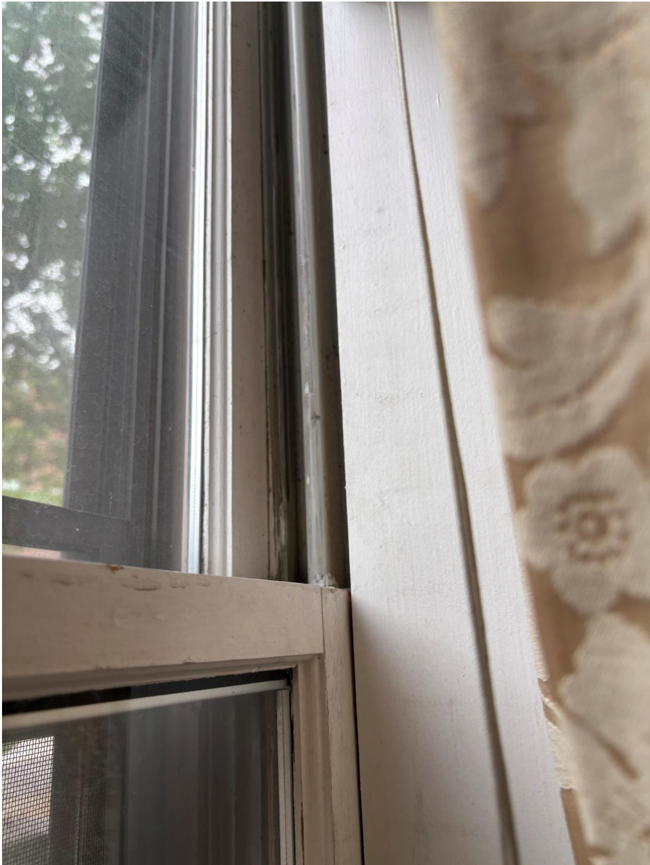
WINDOW 1 NON ORIGINAL JAMBS
