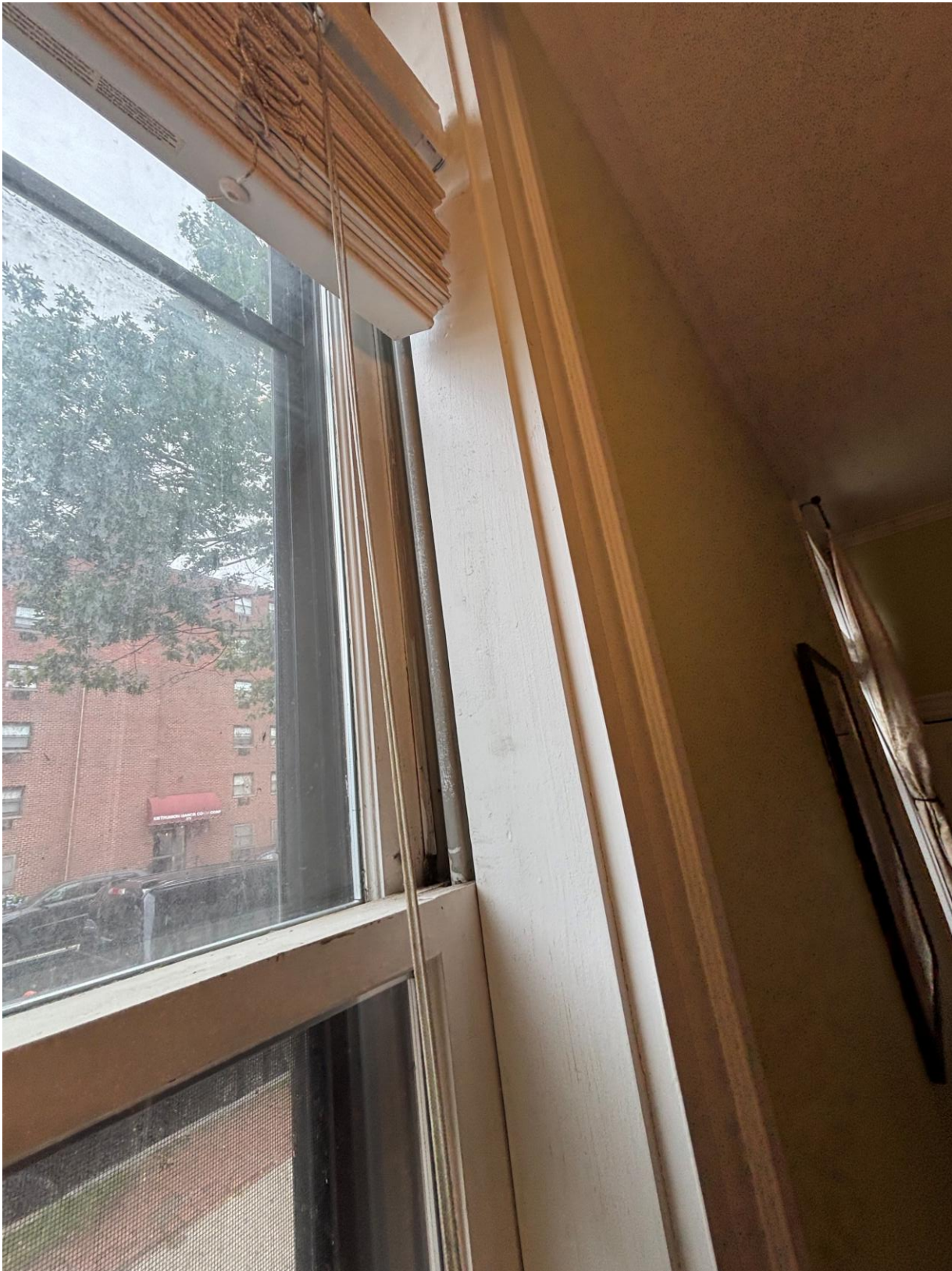
WINDOW 2 NON ORIGINAL JAMBS
