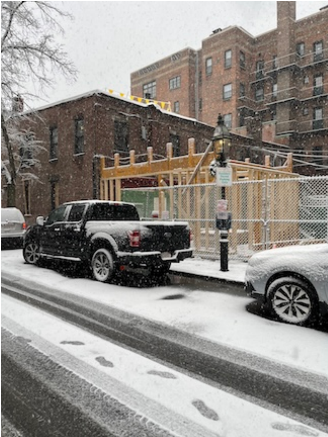
Framing of Replacement One-Story Addition in Progress at Brimmer Street (12/20/2024). (Note: Vertical Posts Support Parapet and will be Concealed by Clapboards.) See Narrative and Drawings for Location of Two Proposed 3.5" Diameter Cameras.
