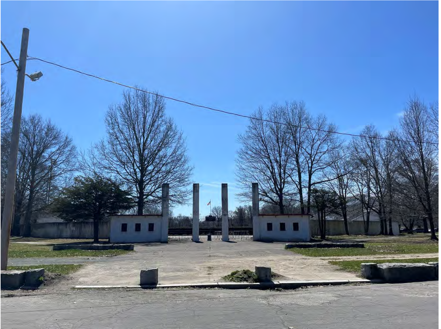
Photo 2. Image of the northern side of the existing infrastructure. Trees included in this assessment were on the right side of the entrance. Trees on the left side of this entrance were investigated in December 2023 with Crowley Cotrell.
