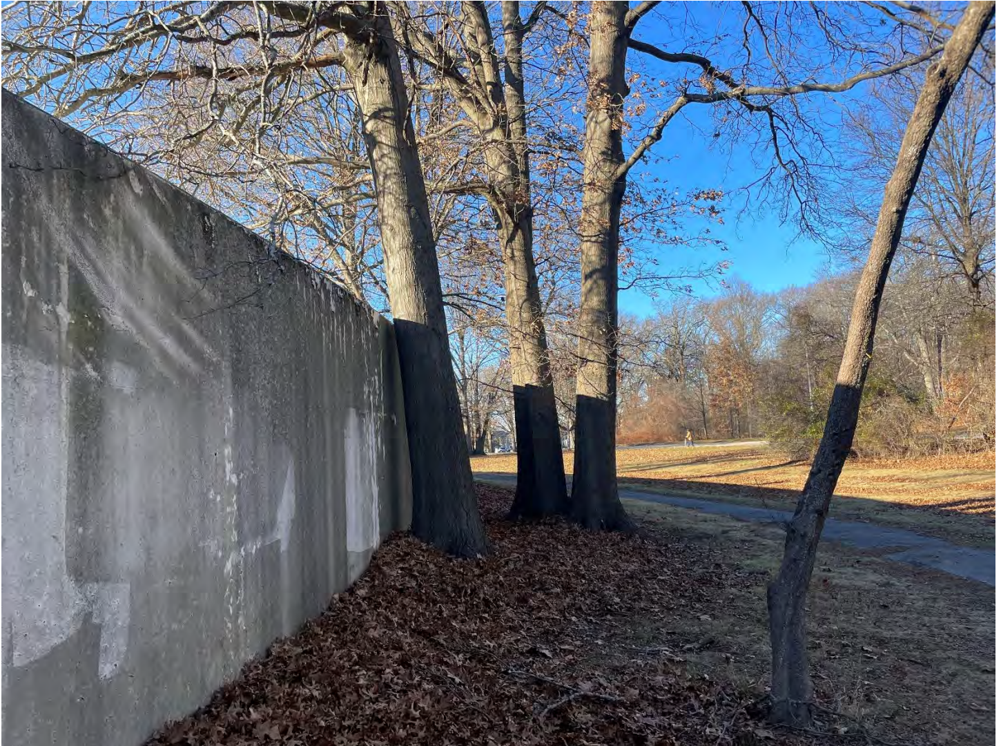
Photo 3. Image focusing on Trees 10, 11, and 12. These trees are located very close to the existing wall. Tree 12 was observed very close to touching the existing wall.
