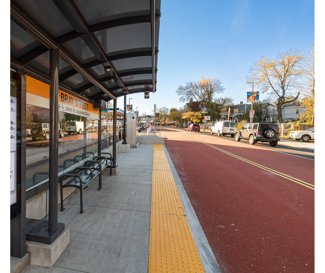
Tactile Warning Strip
