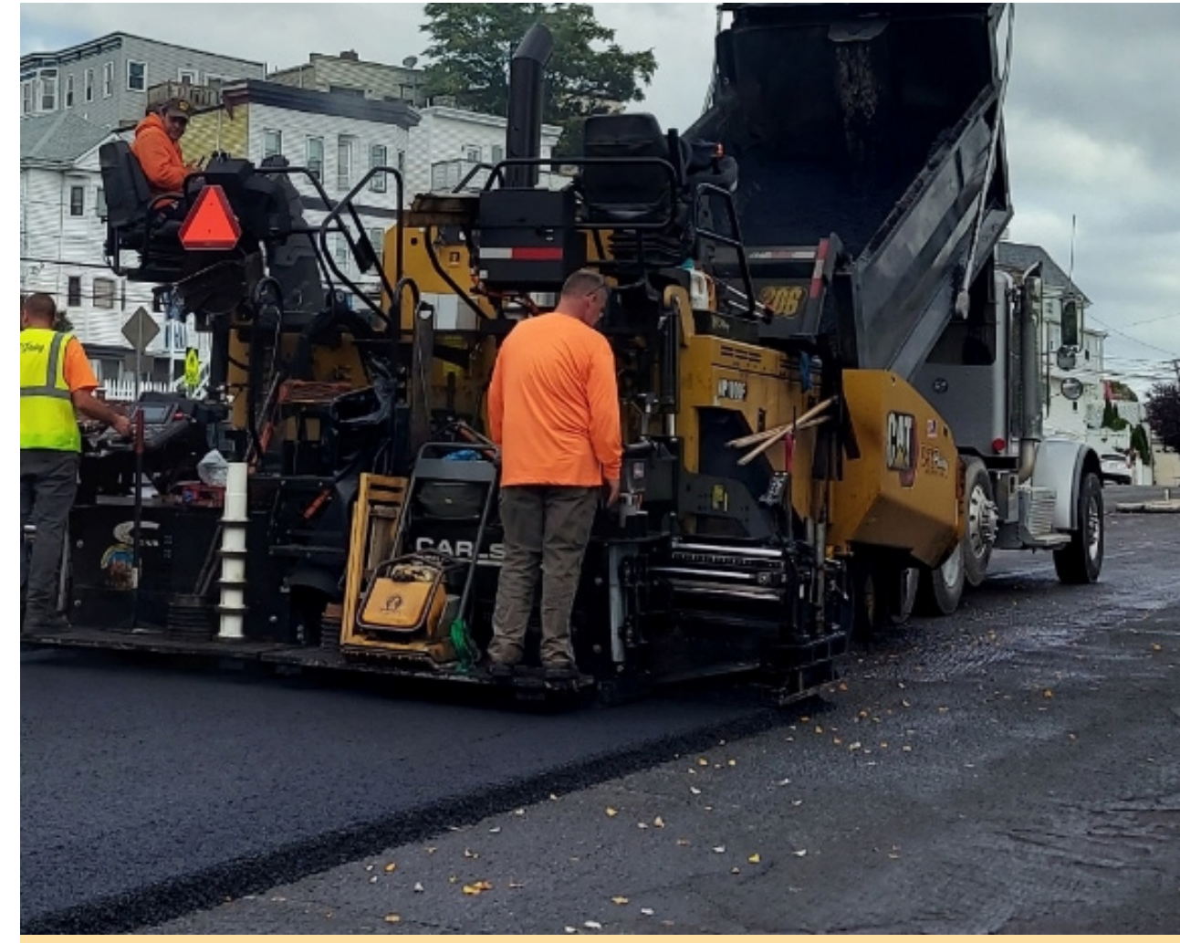
Repaving damaged sections of roadway
