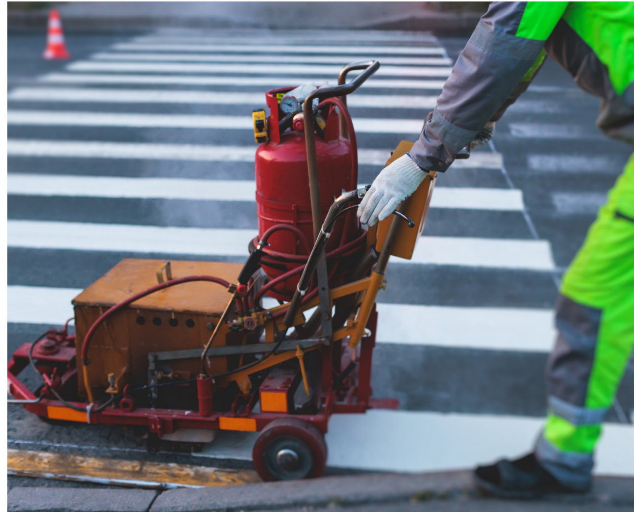
Refreshing crosswalks and pavement markings
