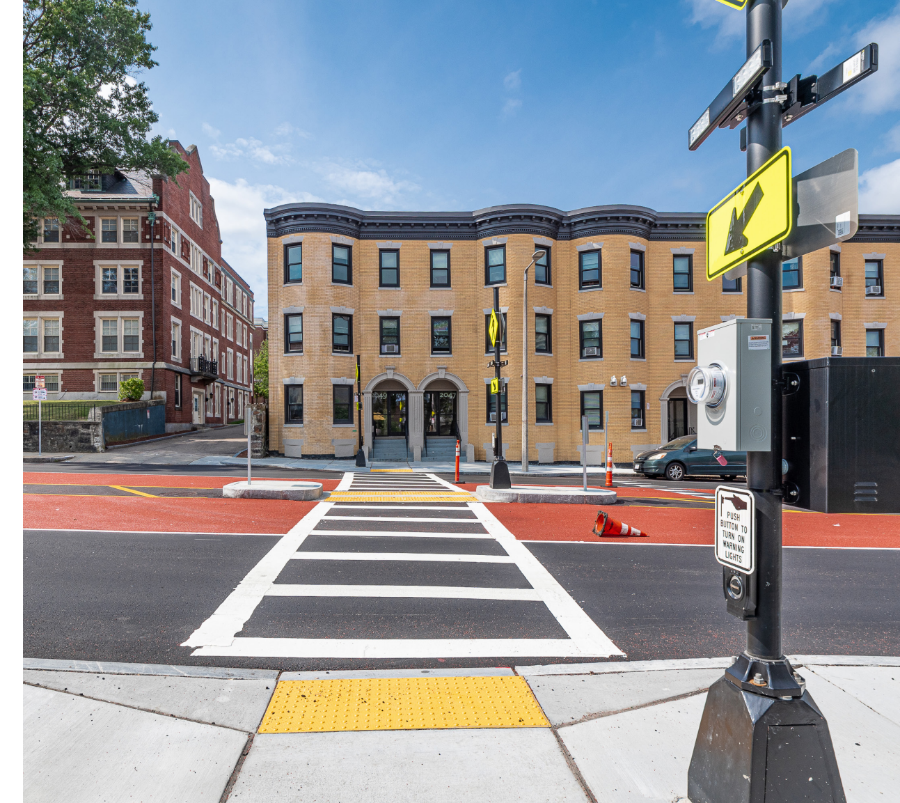
Pedestrian Crossing Refuges
