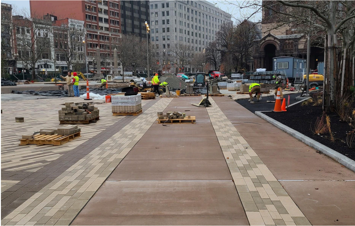
Standing at the corner of St. James and Dartmouth St., a view of the pavers along walkways and in the plaza, to the left. At the time of writing this report, the contractor has completed more of the plaza - but still not enough to open on 12/31/2024 unfortunately.
