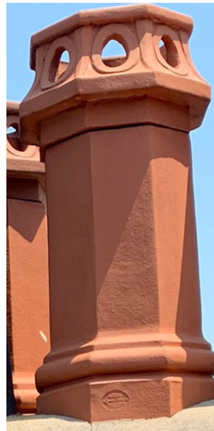
EXISTING CHIMNEY POT TYPE 2
