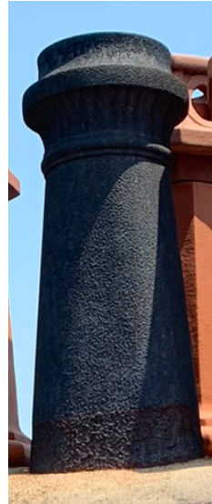
EXISTING CHIMNEY POT TYPE 1
