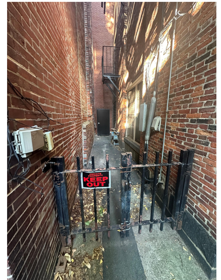
CLOSE UP VIEW OF EXISTING GATE AND LOCATION OF PROPOSED GATE.
