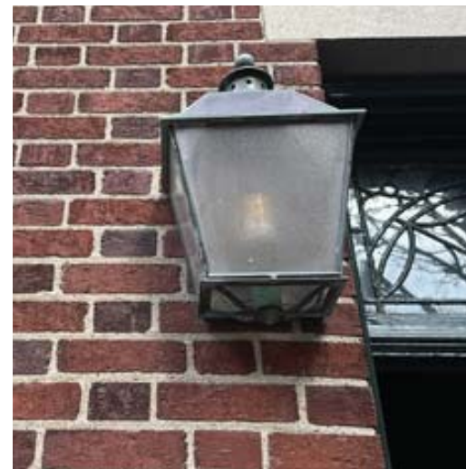
Existing front wall sconce to be repaired and reinstalled
