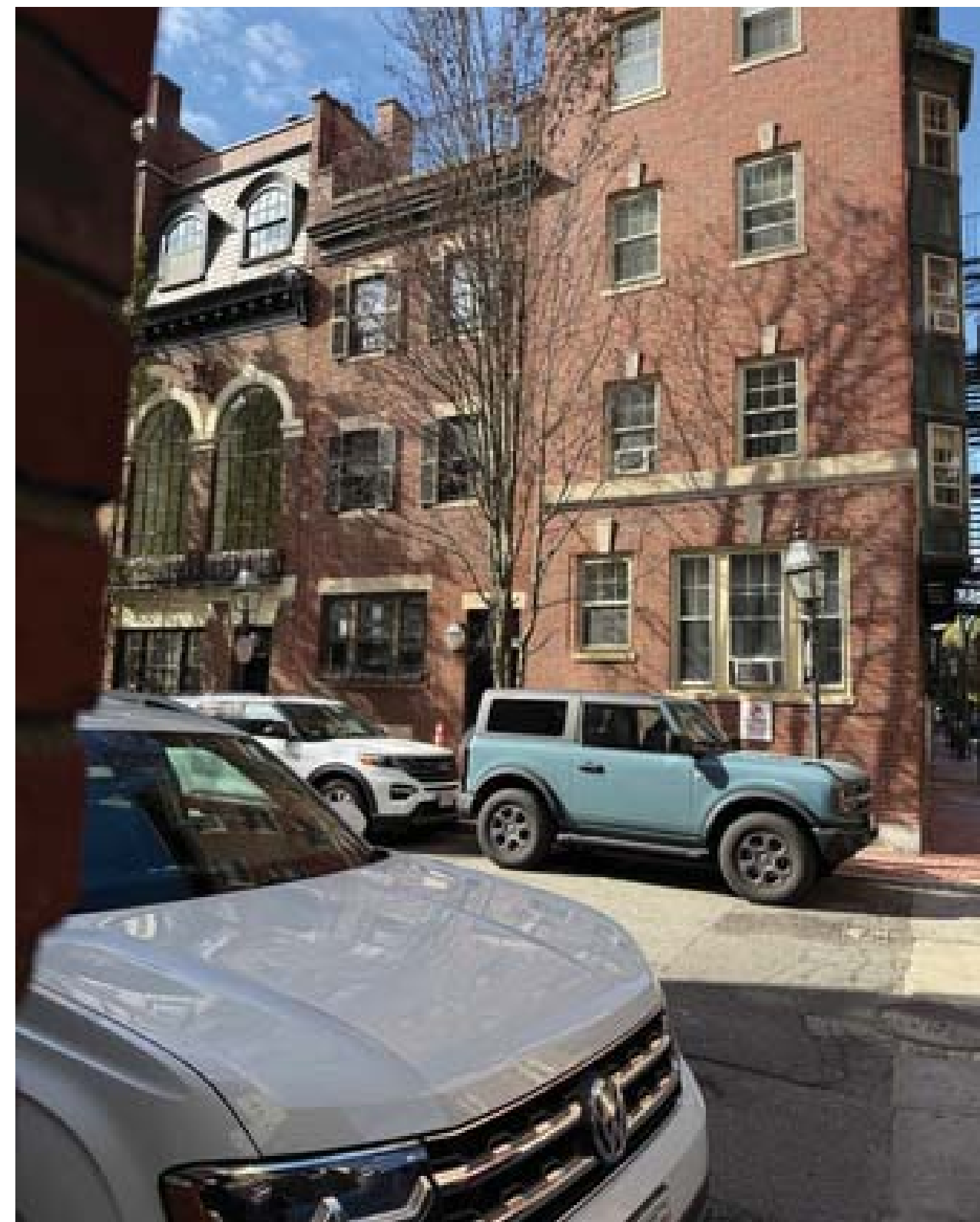
Existing Condition Front (photo taken from River Street)
