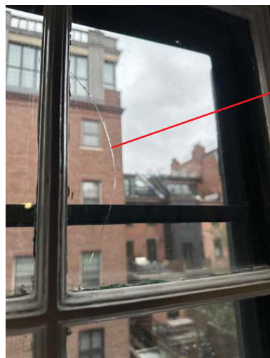
Repair to muntins and replace glass with double glazing
