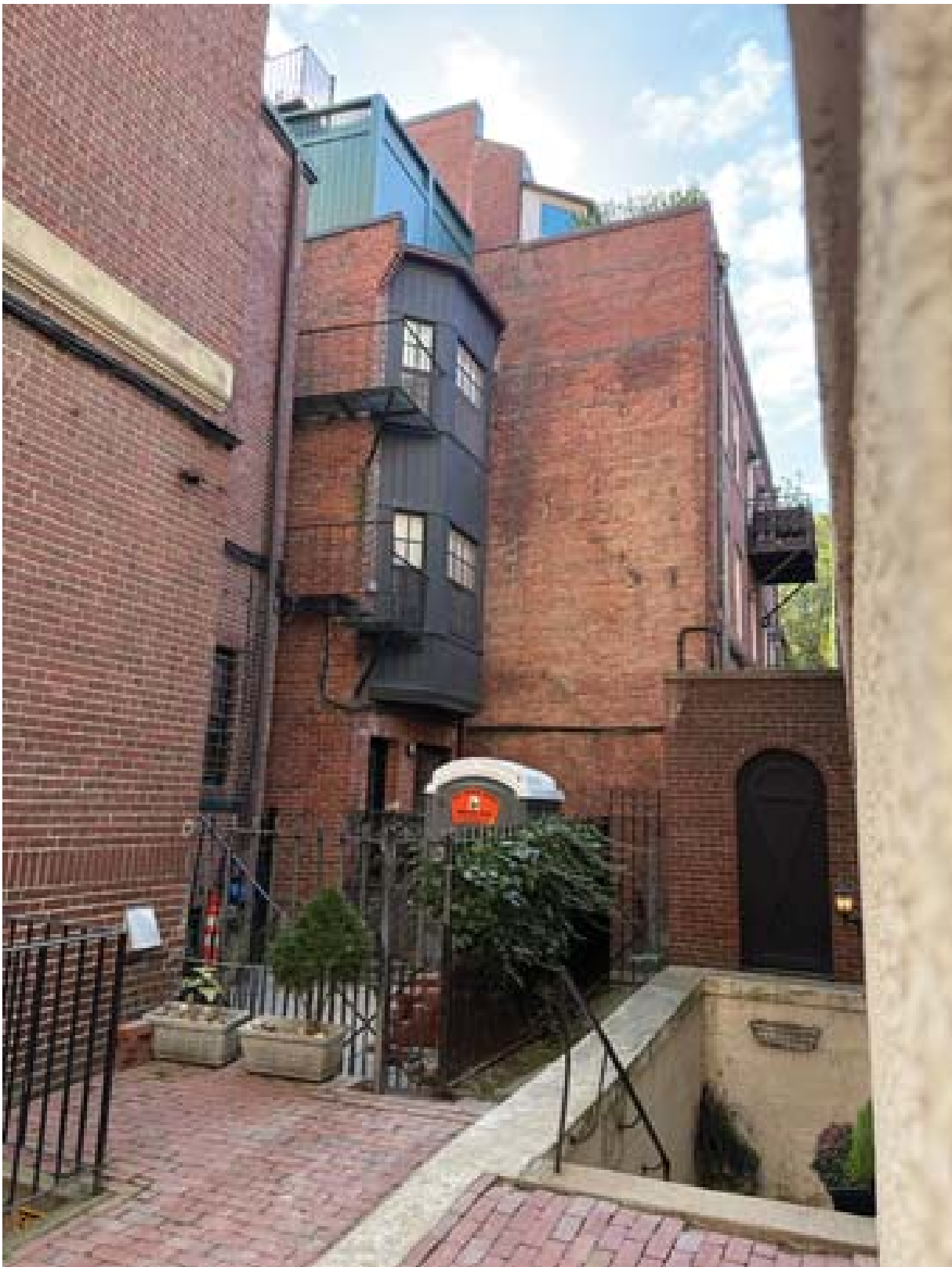
Existing Condition Rear (photo taken from River Street, closest public street)
