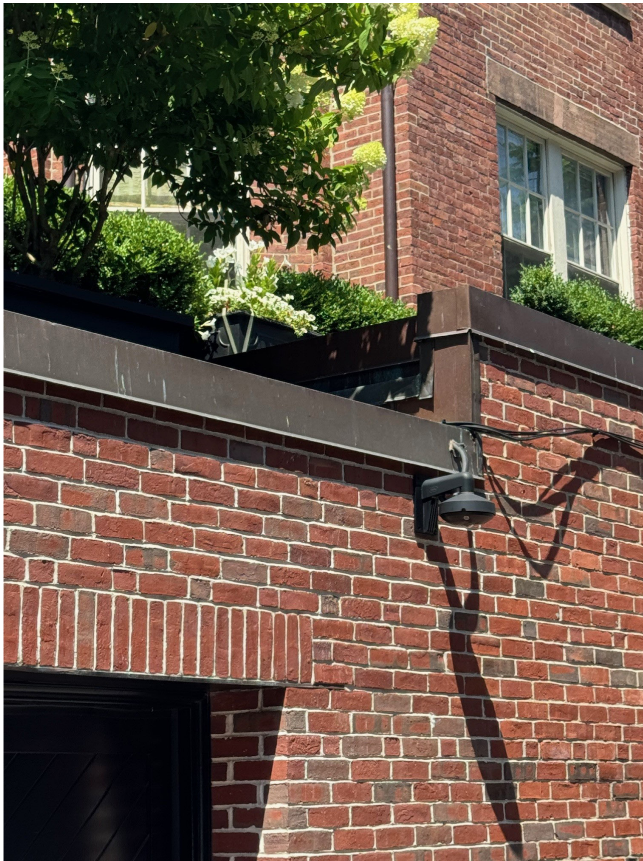
Return Walls on Branch Street
