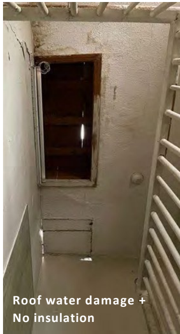
1st floor: damaged ceiling, water leakage
