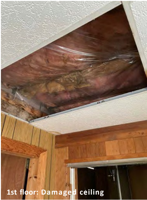
1st floor: damaged ceiling, water leakage
