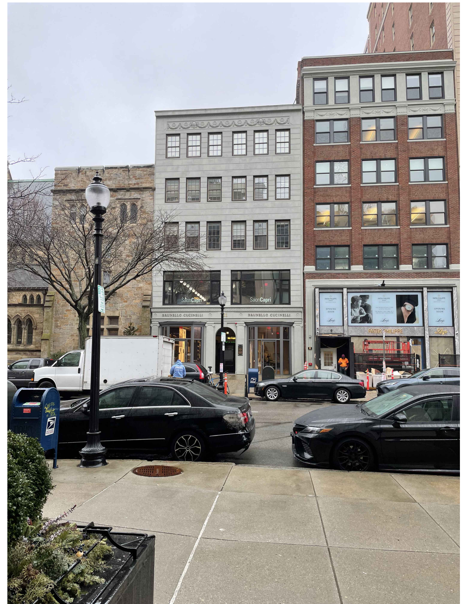
11 NEWBURY STREET - STREET VIEW
