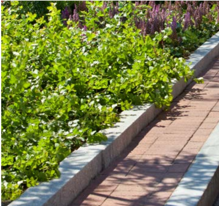
6" Wide granite curb
