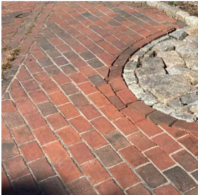
Existing brick paving
