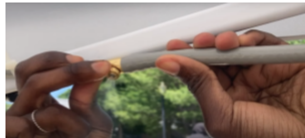
Make sure misting nozzles face inwards
