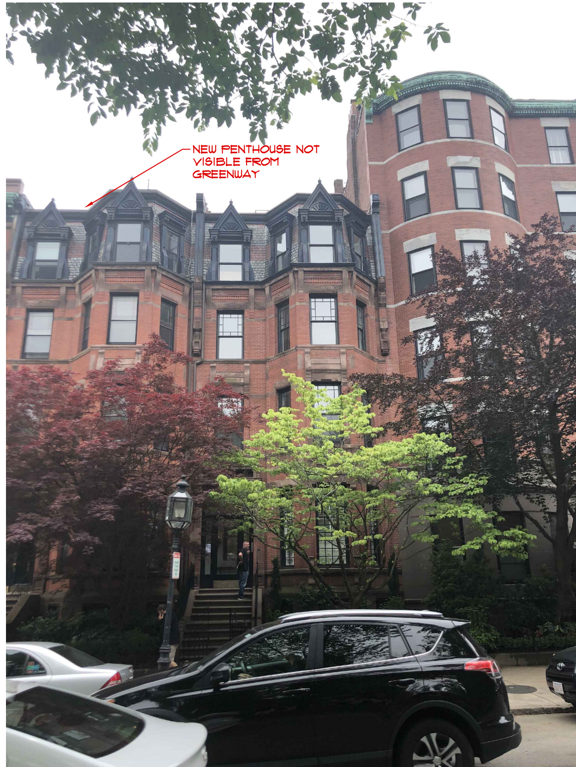
① FRONT EXTERIOR PHOTOGRAPH N.T.S.
