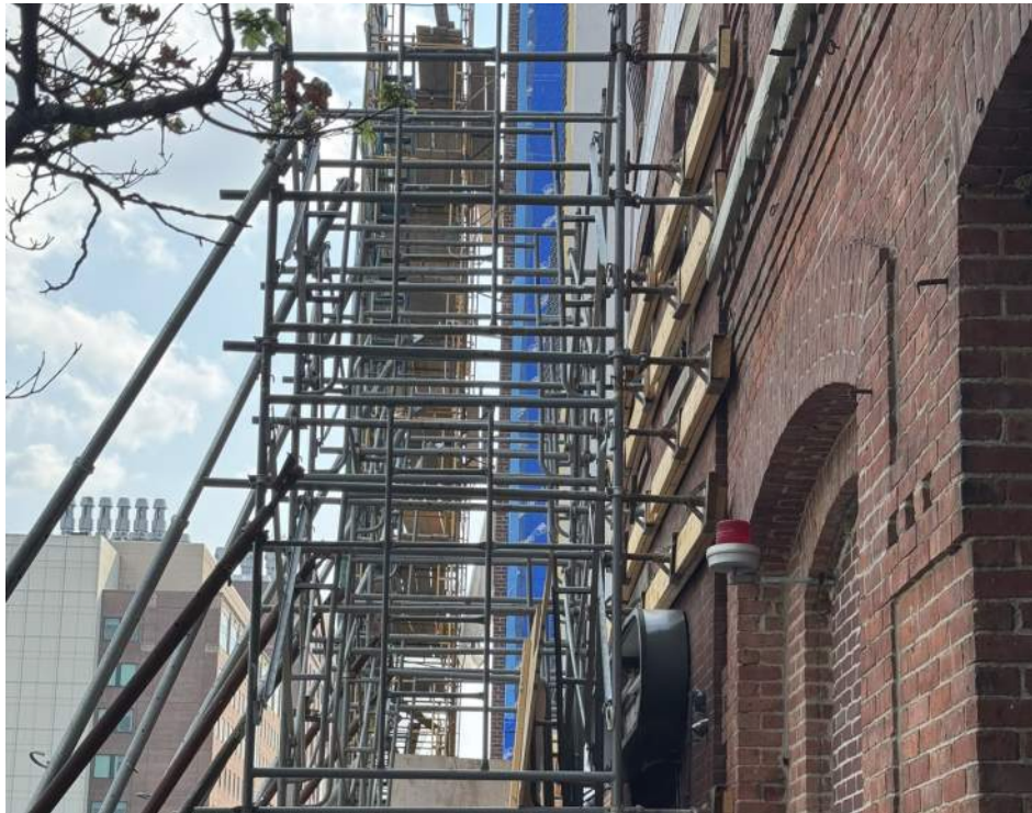
BRACING IN PLACE AGAINST BOWED MASONRY WALL
