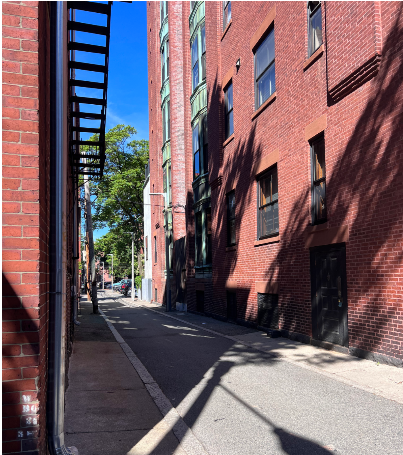
View from Exeter St
