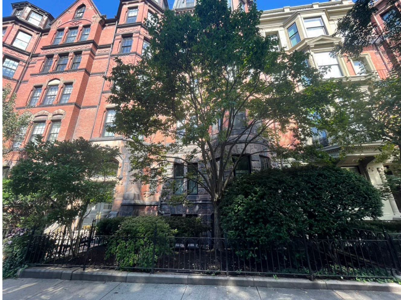
On Commonwealth Avenue, looking straight at the building.
