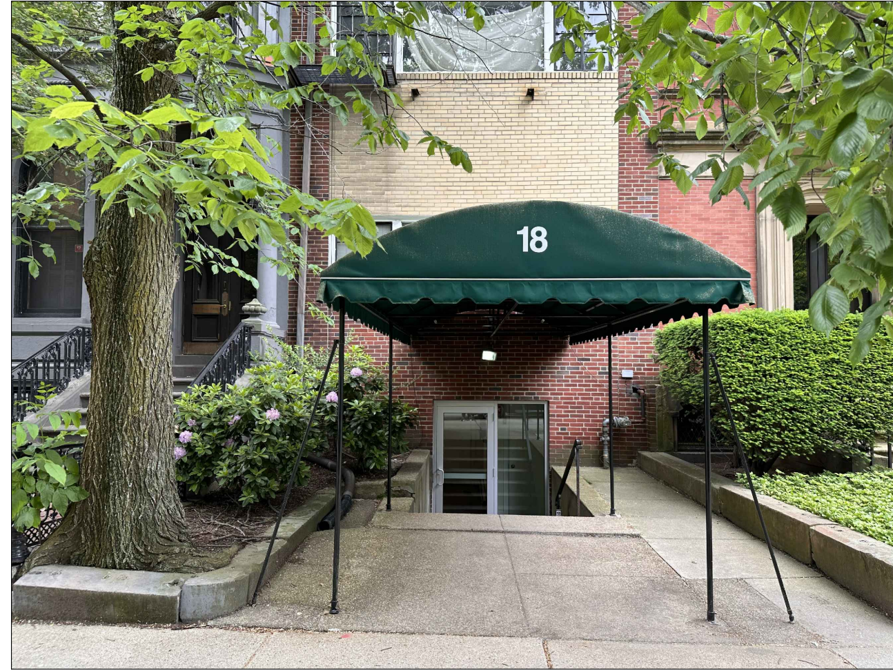
EXISTING FRONT ENTRANCE & GARDEN
