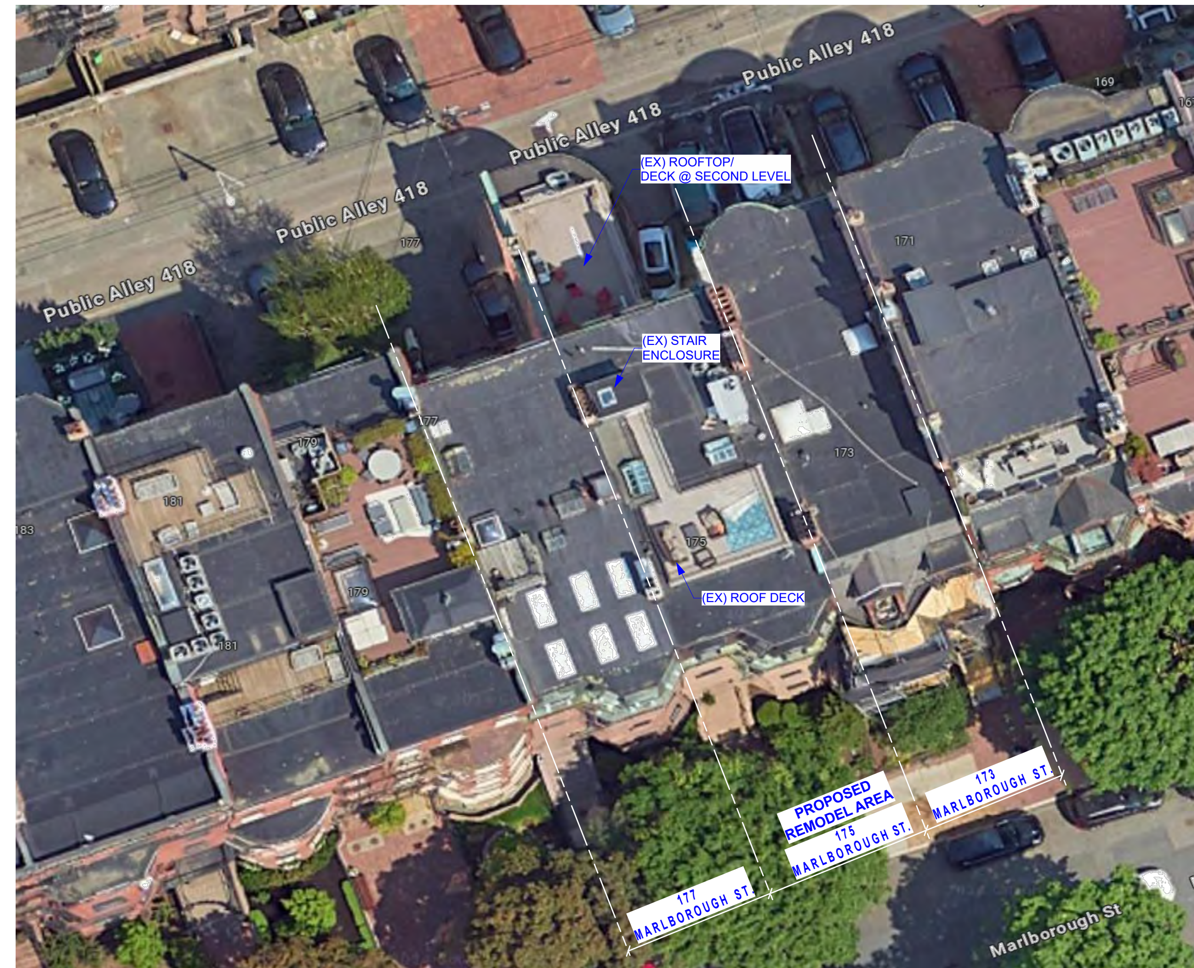
4 PHOTO EXISTING AERIAL ROOFTOP VIEW
