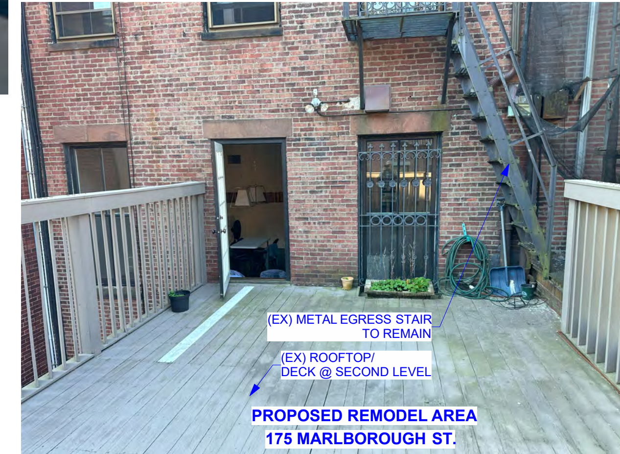
2B EXISTING SECOND LEVEL DECK
