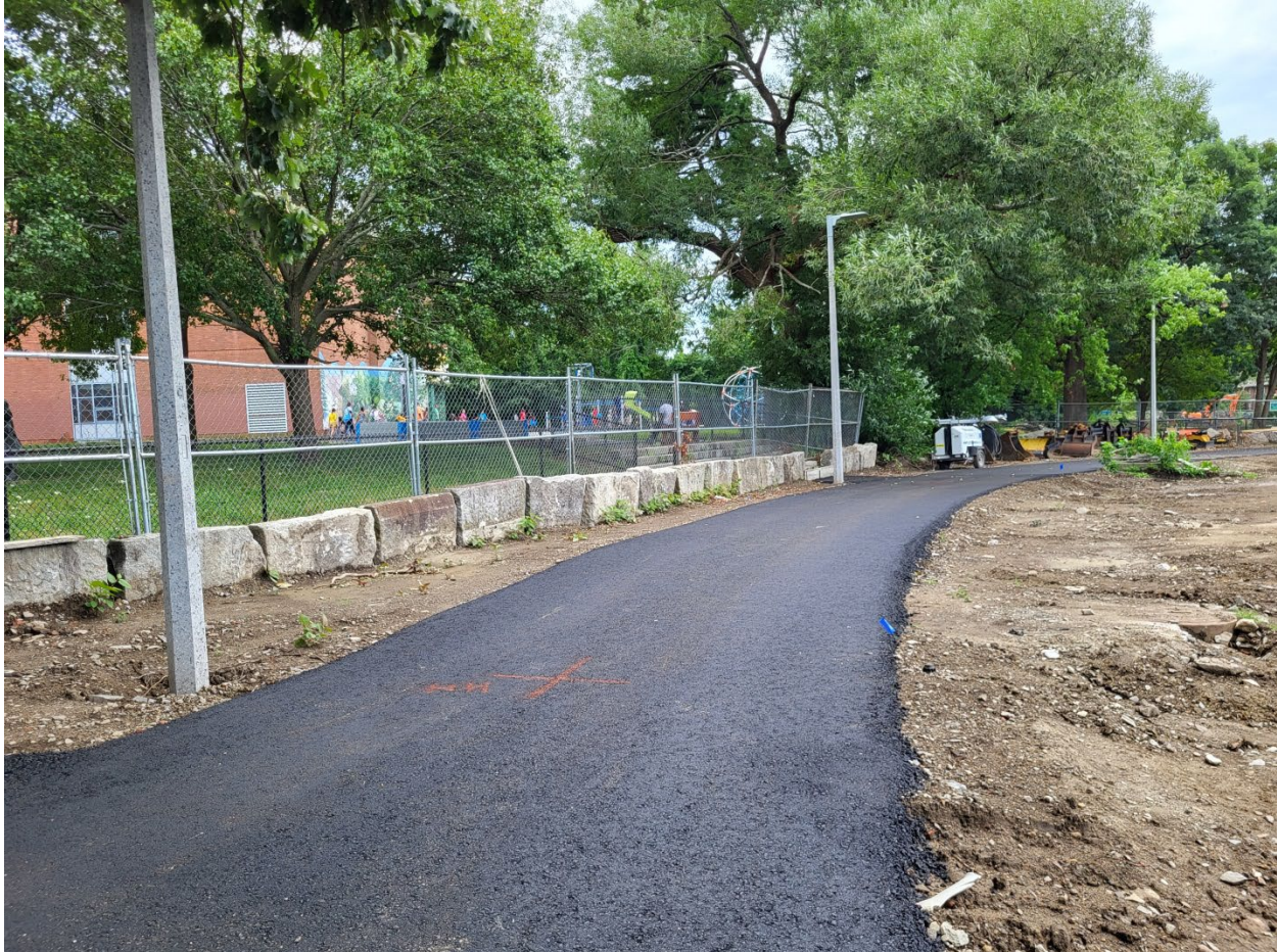
Asphalt base course at the pathways
