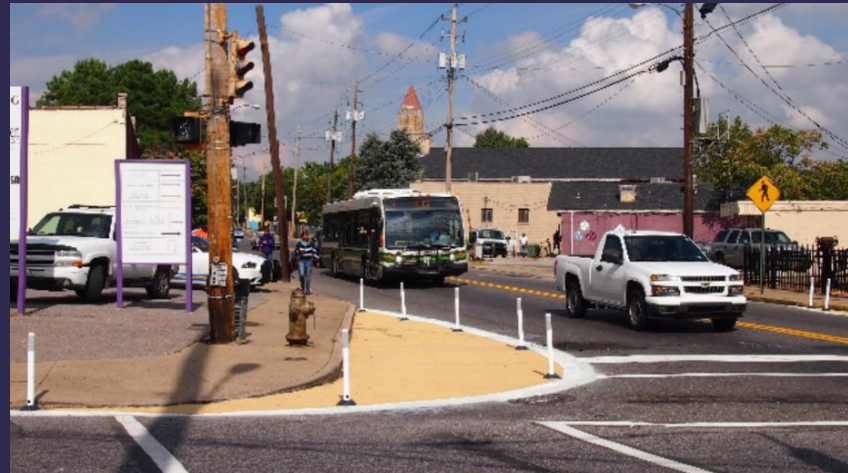
Corner curb extension; Memphis, TN
