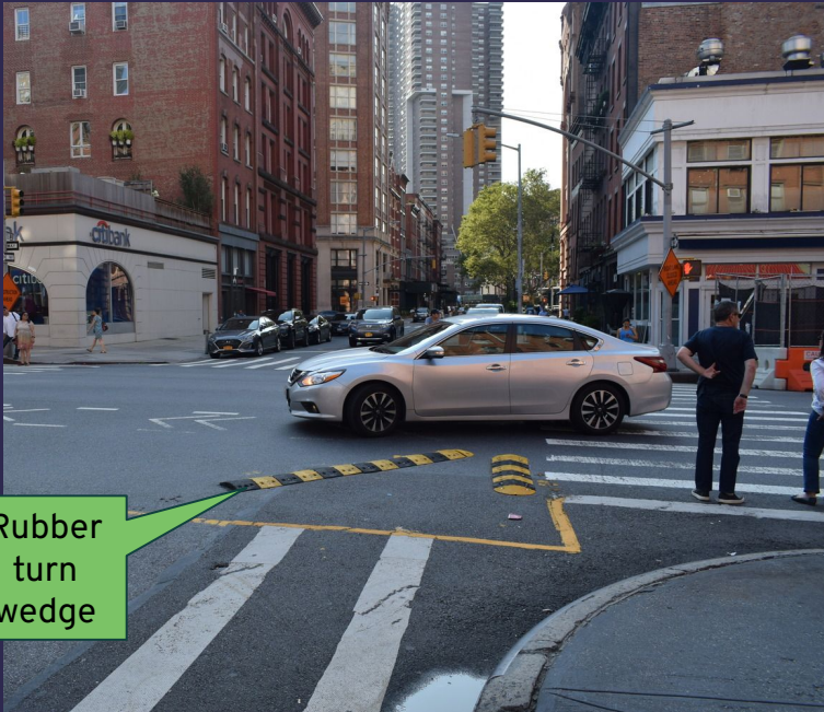
Reducing curb radii with a "turn wedge", NYC, NY
