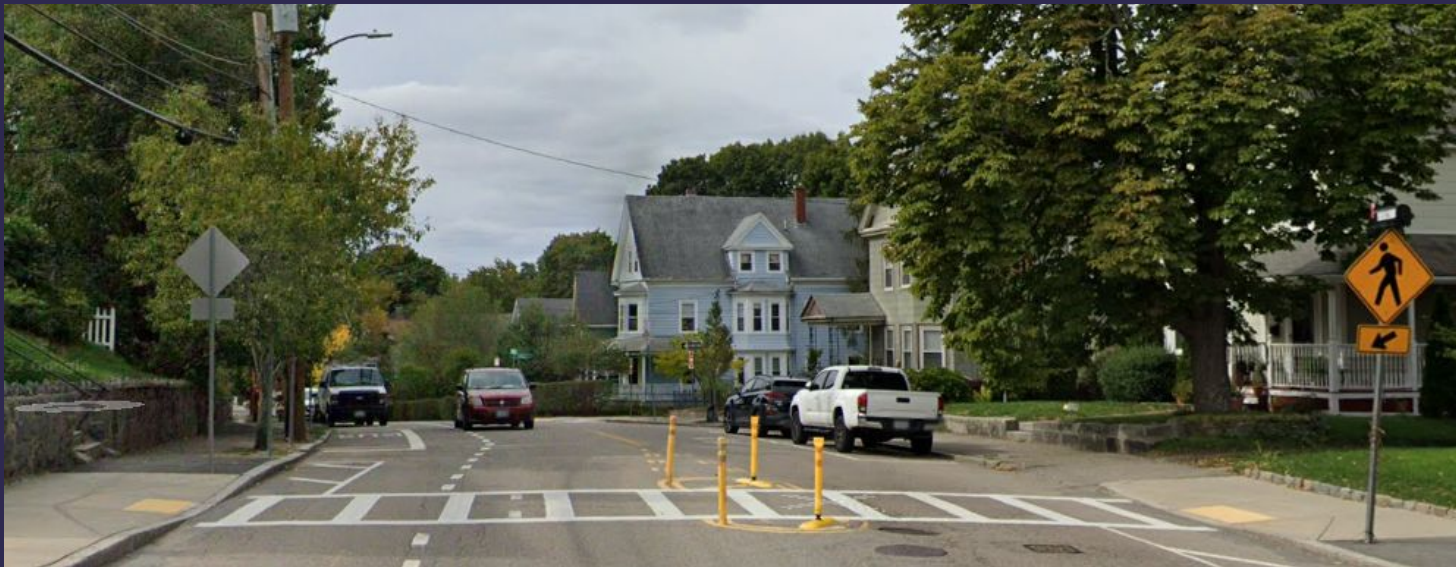
Painted median island with posts on Walter St, Roslindale, MA
