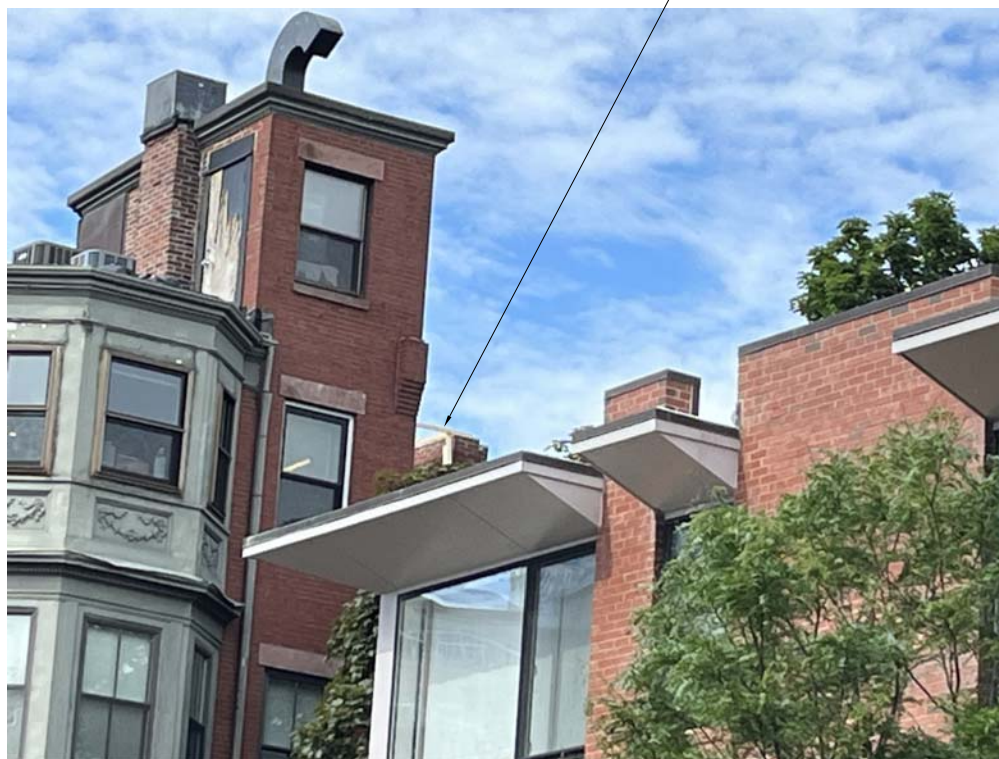
LONG VIEW FROM CLARENDON SOUTH (DETAIL)
