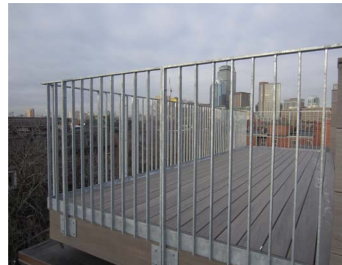
EXAMPLE GALVANIZED STEEL RAIL (GREY) TO BLEND WITH SKY. PROPOSED AS ALTERNATE TO BLACK RAIL IN EXCHANGE FOR PARTIAL VISIBILITY.
