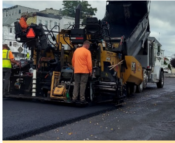
Repaving damaged sections of roadway
