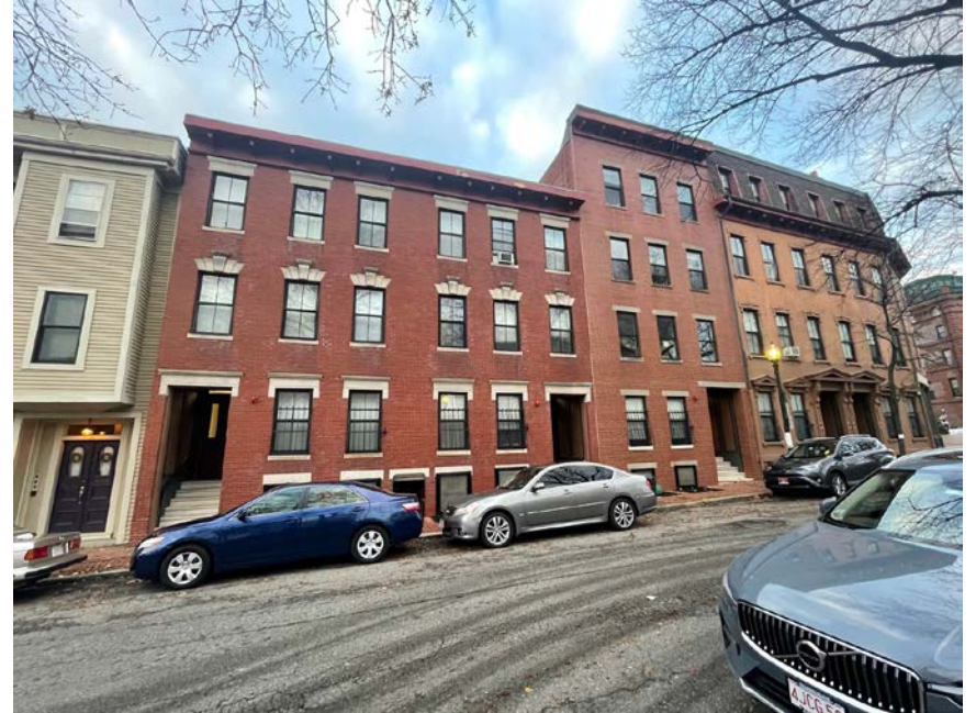
On Dudley St Across From Site
