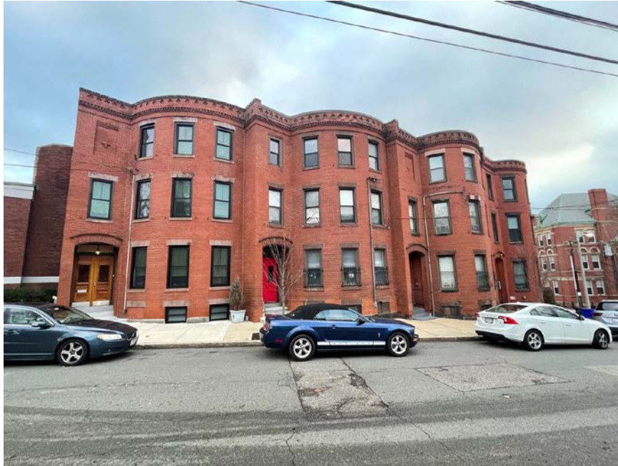
On Kenilworth Next to Site
