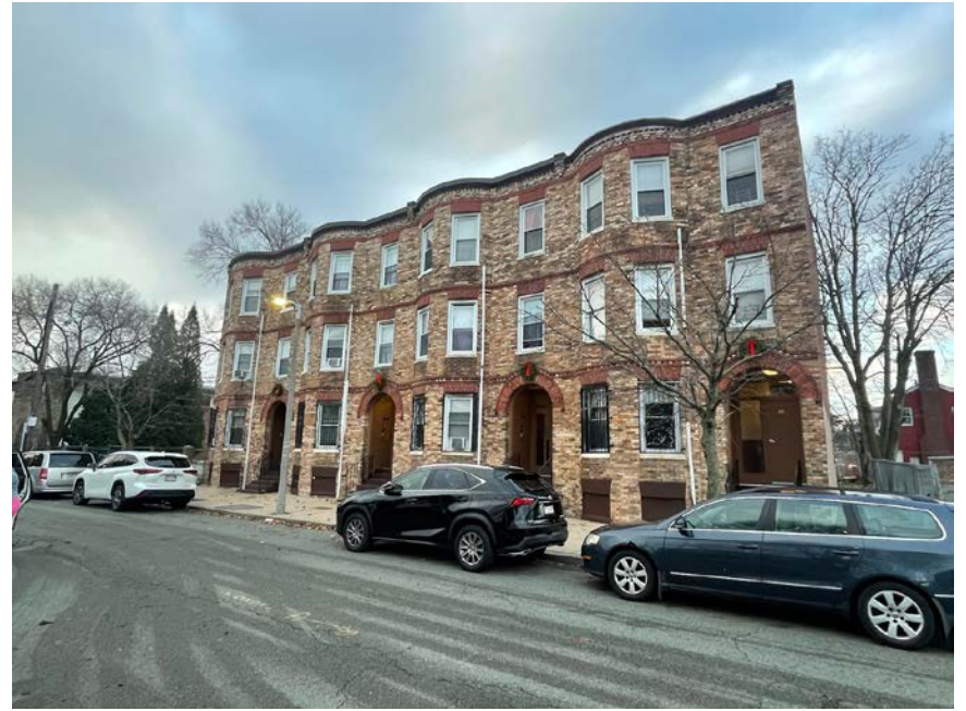
Across Kenilworth from Site
