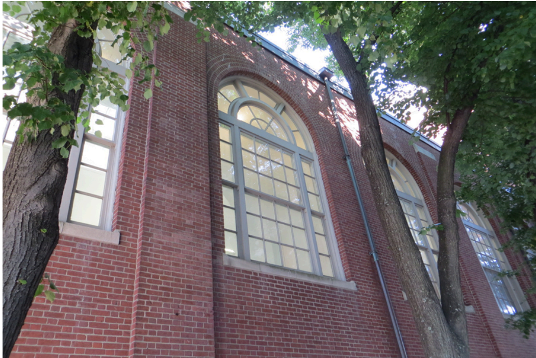
Figure 10. Windows on the one-story section of east elevation (looking west). June 2016.
