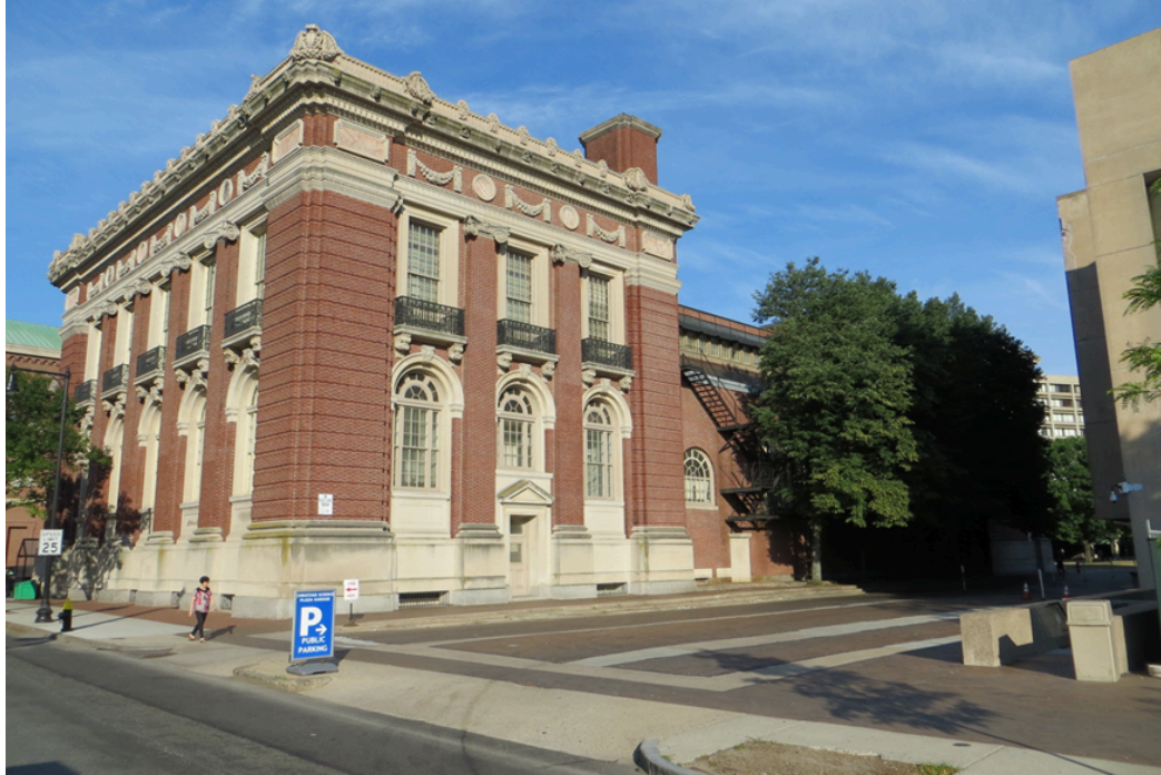
Figure 3. South (facing Huntington Avenue) and east (facing Christian Science Center complex) façades of Horticultural Hall (looking northwest). June 2016.
