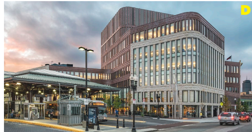
2300 WASHINGTON ST. - BRUCE C. BOLLING MUNICIPAL BUILDING
