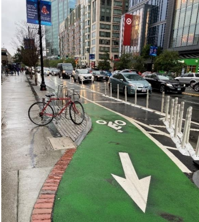
Separated bike lane with flex posts Location: Boylston Street, Fenway
