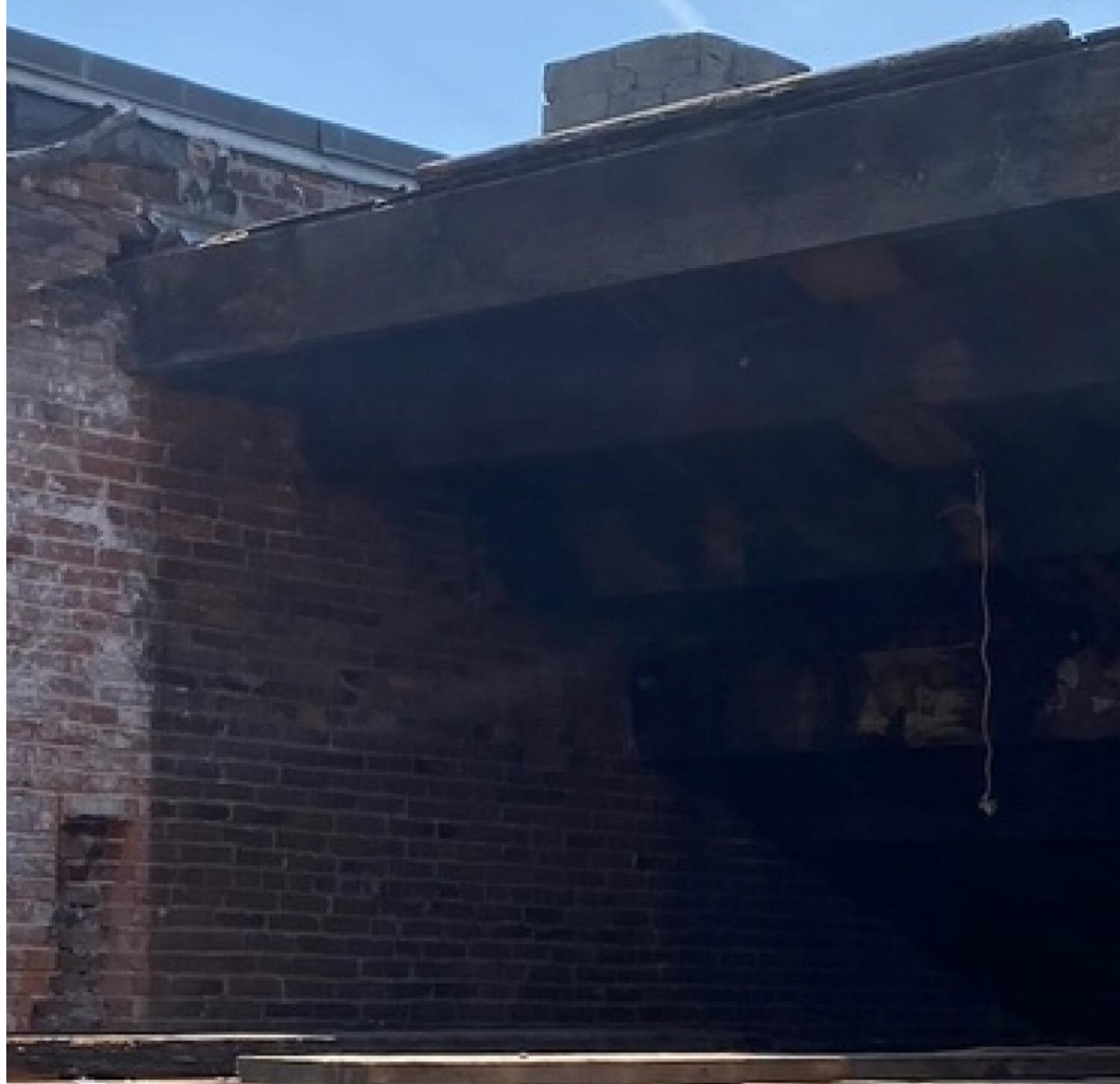
IMAGE OF THE EXISTING RIDGE BEAM
