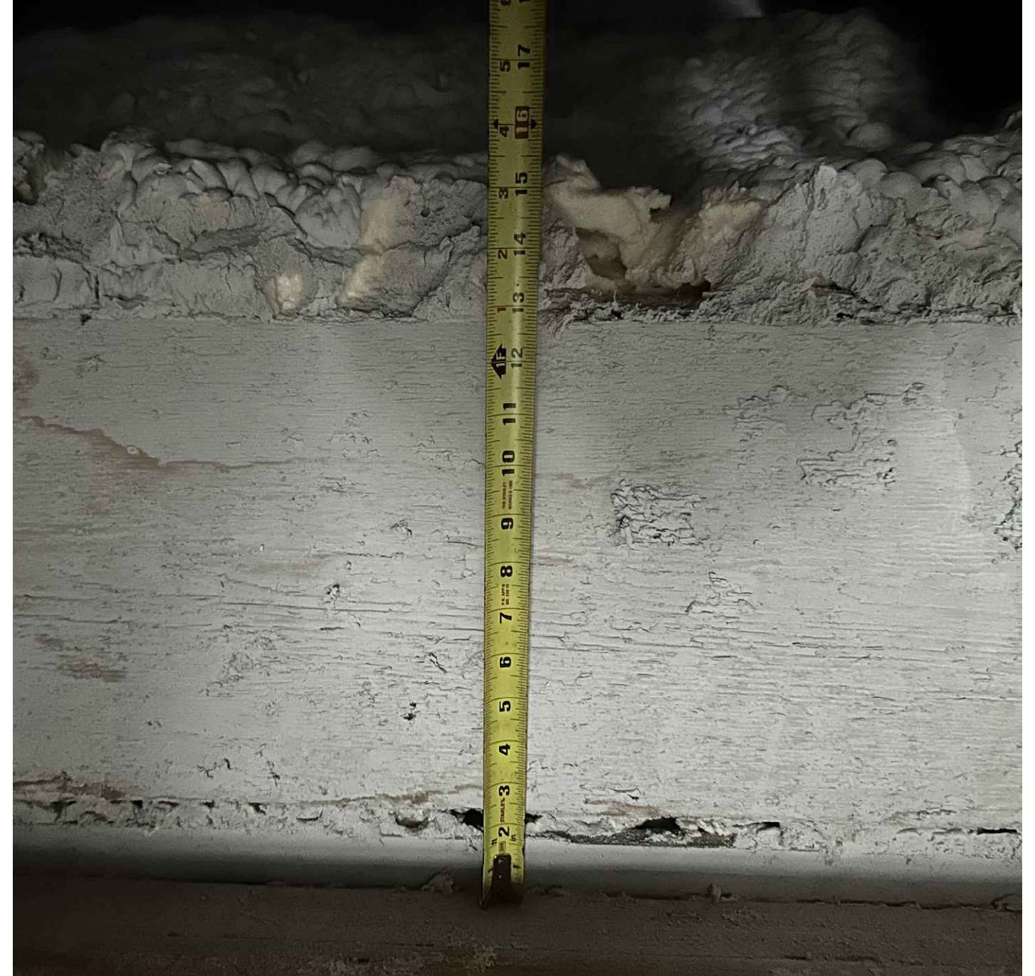
IMAGE OF THE EXISTING RIDGE BEAM IN INSULATED ATTICE SPACE
