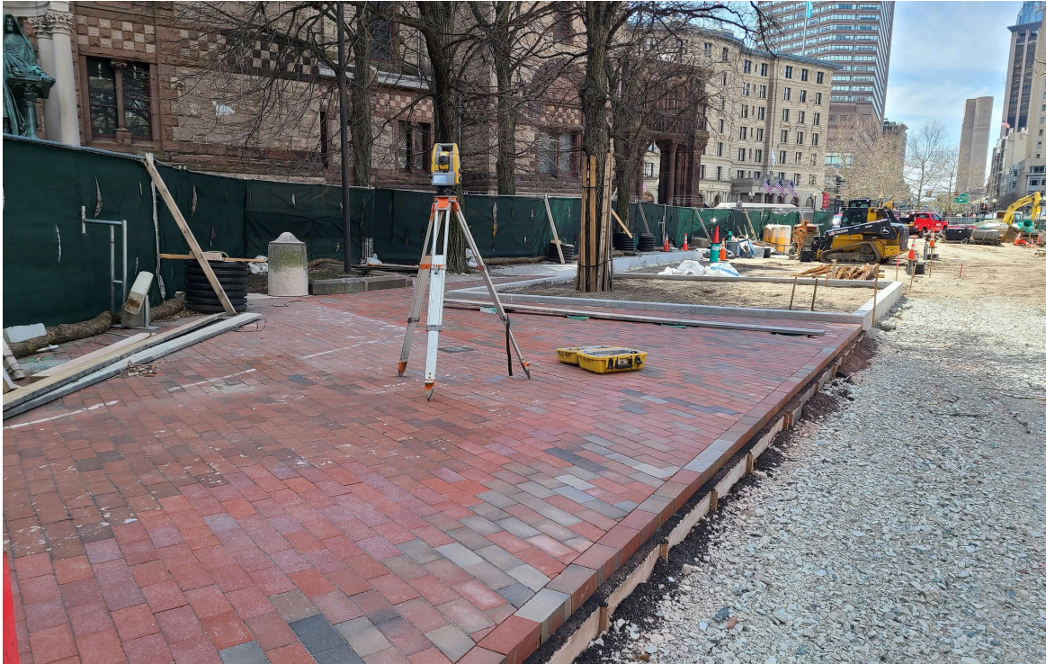
New brick pavement north of Trinity Church is being installed. Concrete walkway next!
