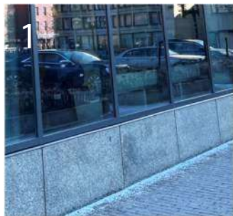
1 Granite Wall Base to Match Existing
