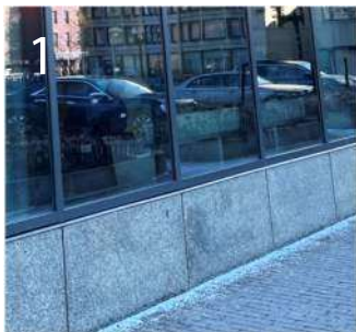
1 Granite Wall Base to Match Existing
