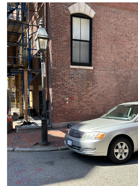
EXISTING VIEW OF F.D.C. WITH FIRE BELL LOCATION AS PROPOSED BY FIRE DEPARTMENT
