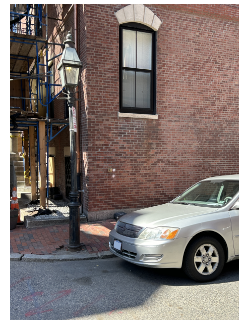
EXISTING VIEW OF F.D.C. AT I OTIS PLACE FROM & BRIMMER STREET
