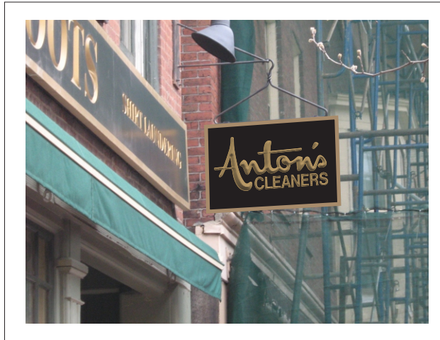
EXISTING CONDITIONS * NOTE - COAT HANGER SHAPED BRACKET *
